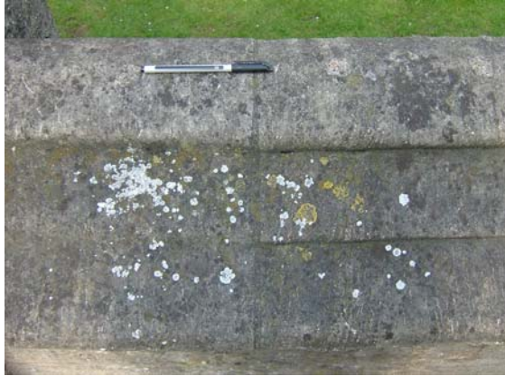
A view of the variety of lichens that can be found lower down on the same string course.
