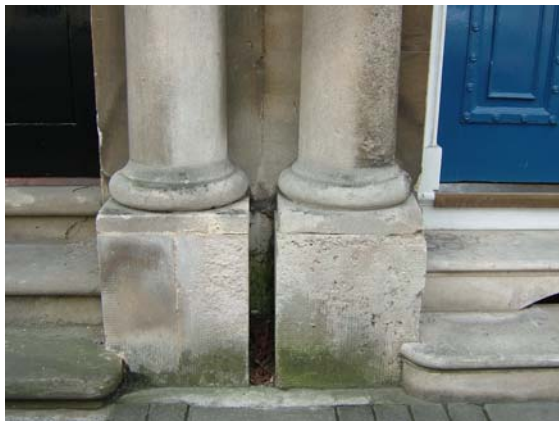
Left hand column base shows roughening due to salt weathering on right hand side, Beaumont Street.
