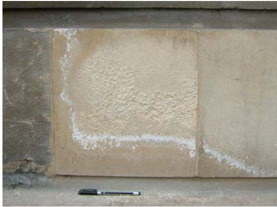
Salt tide and roughened flaking surface caused by salt weathering, Beaumont Street.
