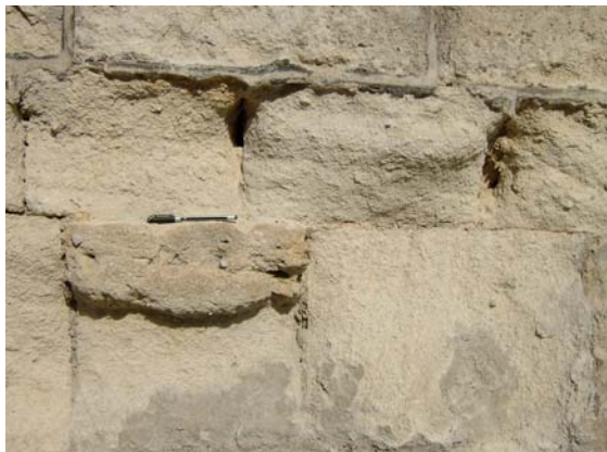
Close-up of cavernous weathering on this recently cleaned part of the boundary wall.
