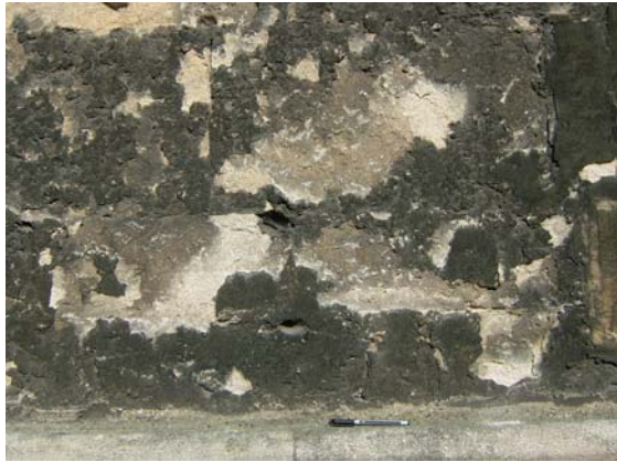
Exfoliating framboidal gypsum crust on Headington freestone also above the plinth at the Bodleian Library.
