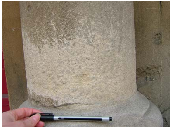
Pitting, roughened texture at base of column – possibly caused by salt weathering, Beaumont Street.
