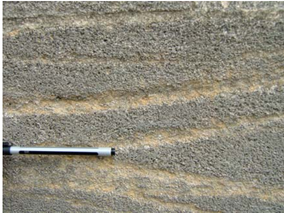
Dissolution focused along bedding planes, St. John's College.
