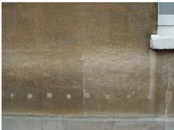
Scratch marks on Bath stone ashlar from bicycle handlebars, Beaumont Street.
