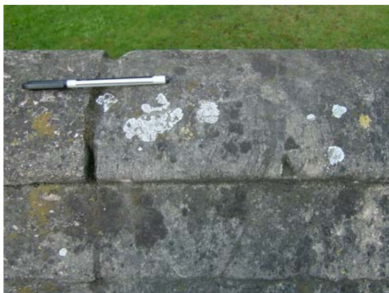
Lichens growing on a south-facing string course at Magdalen College on High Street.
