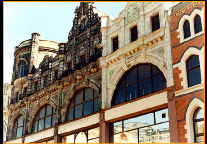
Buildings in Belfast City Centre. Façades which illustrate the contrast between soiled and cleaned buildings.
