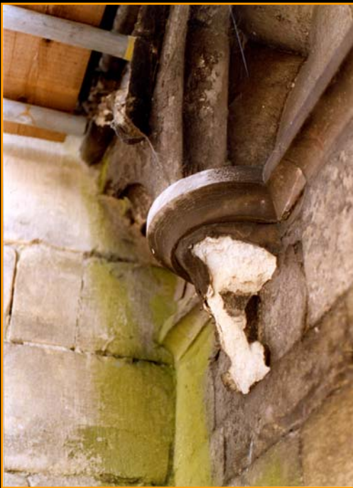
York Minster. This section of stonework shows differential weathering of original Tadcaster/Huddleston limestone and replacement Ketton stone, introduced as part of restoration work in the early 20 th Century. Ironically, it is the replacement Ketton stone that is showing the most serious damage.
