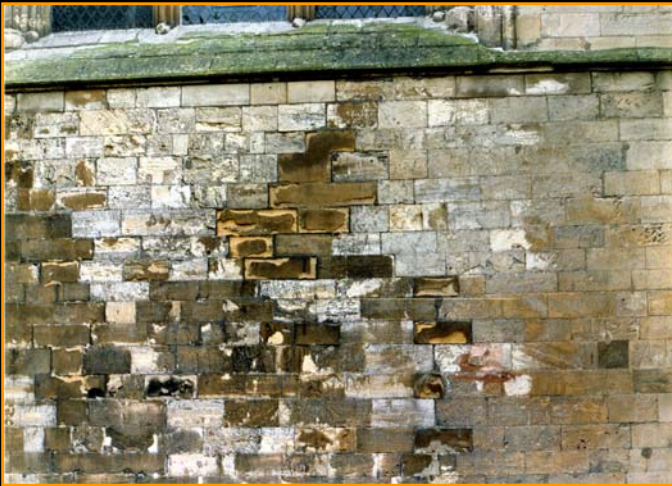
York Minster. This section of stonework shows differential weathering of original Tadcaster/Huddleston limestone and replacement Ketton stone, introduced as part of restoration work in the early 20 th Century. Ironically, it is the replacement Ketton stone that is showing the most serious damage.
