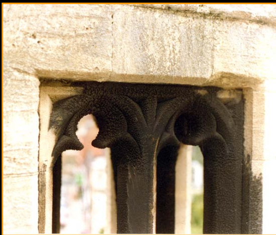
Gloucester Cathedral. Extensive black crust development on Paineswick Stone in an area protected from rain.
