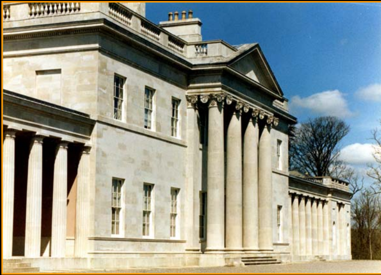
Castle Coole, Co. Fermanagh. Despite its rural location, parts of the building show evidence of significant solution and salt weathering of limestone. Castlecoole's proximity to Enniskillen means that it may be exposed to minor concentrations of urban pollutants, but probably receives most salt as wind-blown particulates from the Donegal coastline.
