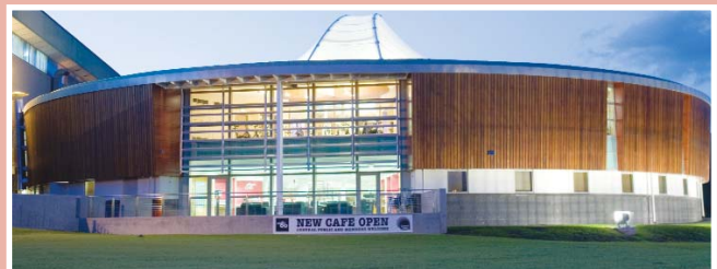
Extension to Physical Education Centre
