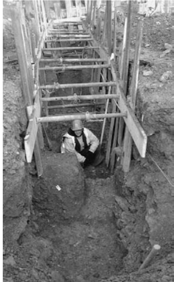
Figure 2.3 Trench with health and safety features
