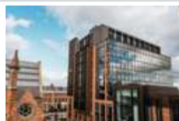
2 The Main Site Tower
