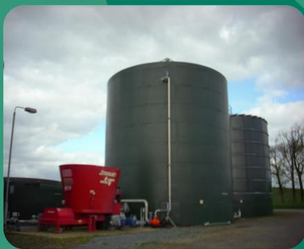
Fig. 1. The mesophilic two-stage anaerobic digester located in Hillsborough (AFBI)
