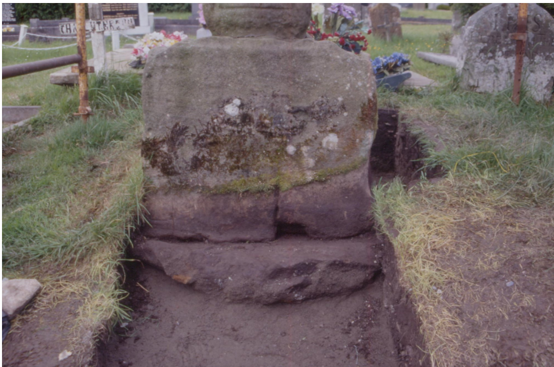
Plate Four: Trench One following the excavation of the humic layer (Context No.2) (looking west).
