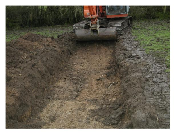
Photo 5: Excavation of Trench 1 showing utilization of toothless "sheugh" bucket.
