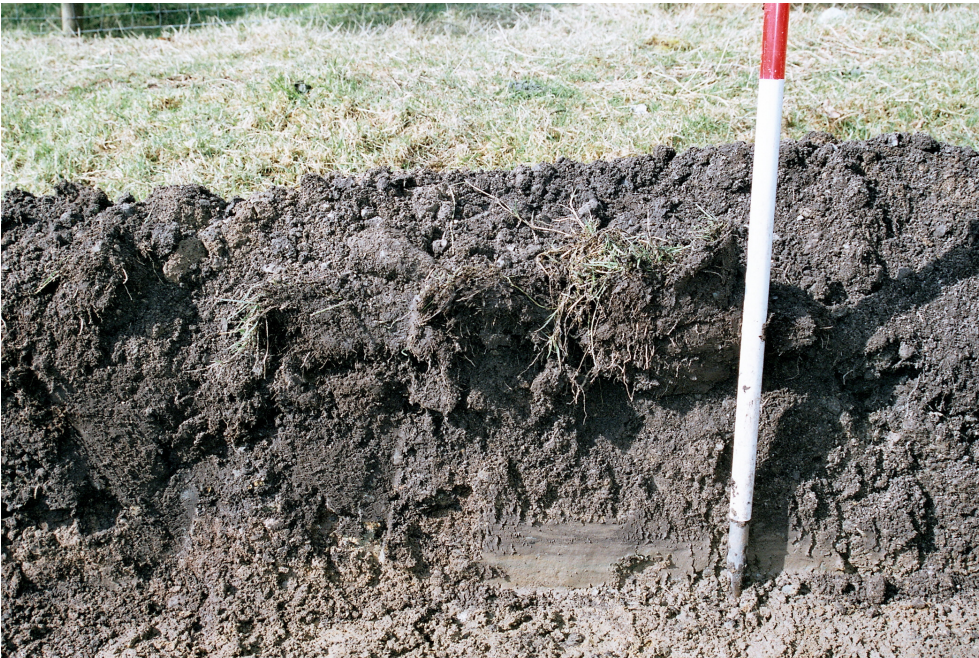
Plate 8: View of east-facing section in Trench D, after excavation to surface of subsoil (C402).
