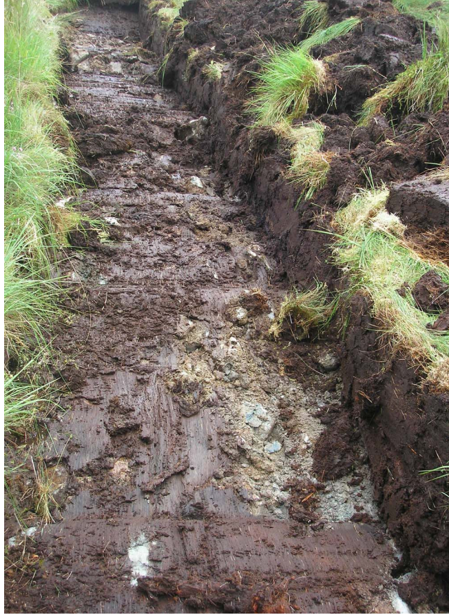
Plate Nine: Trench Three following excavation to subsoil (Context No. 303), looking north-east
