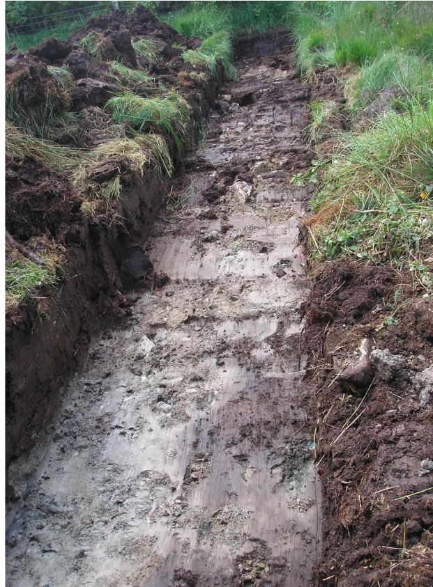
Plate Eleven: Trench Four following excavation to subsoil (Context No. 403), looking south-west
