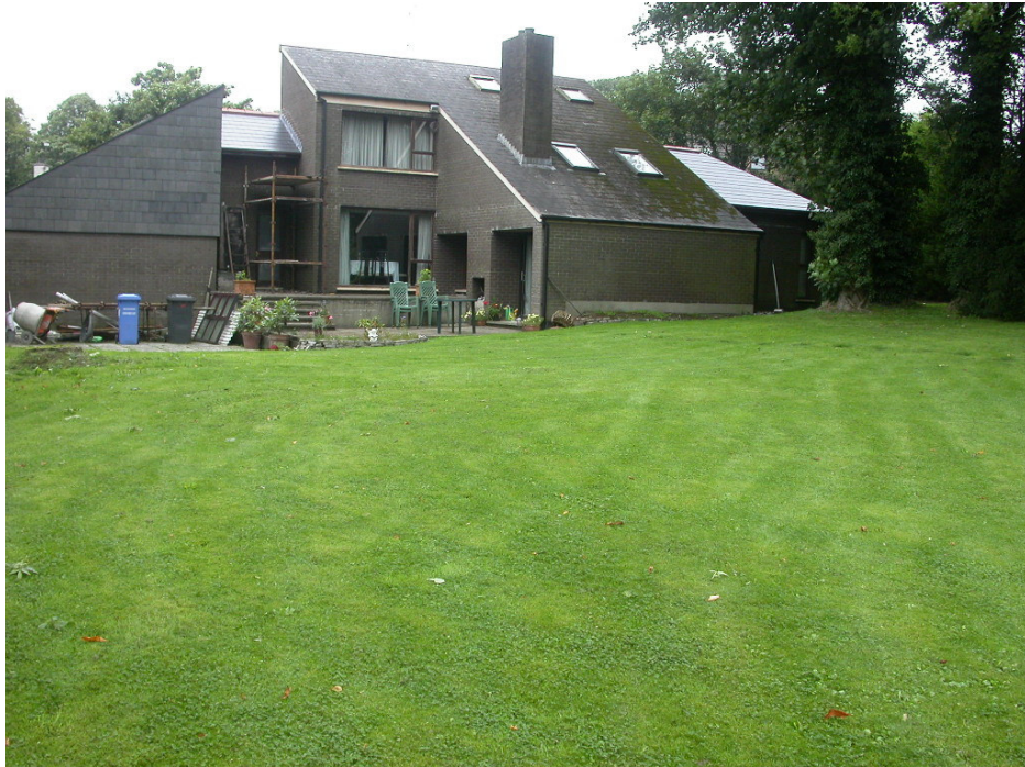
Plate One: Proposed development site, prior to evaluation, looking north
