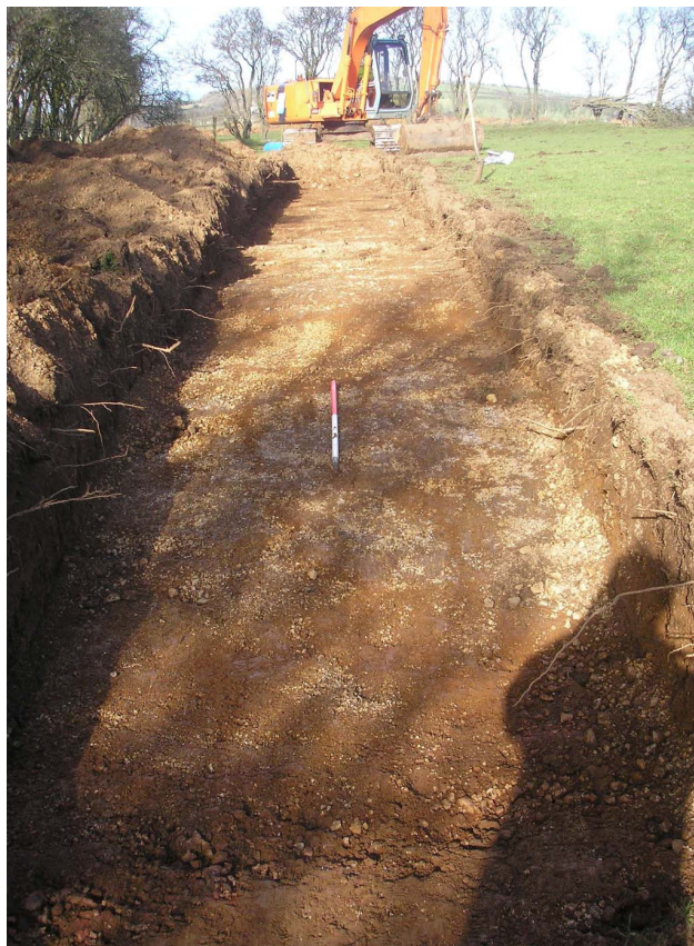
Plate 11: Trench 5 following excavation to subsoil (Context No. 503), looking north.
