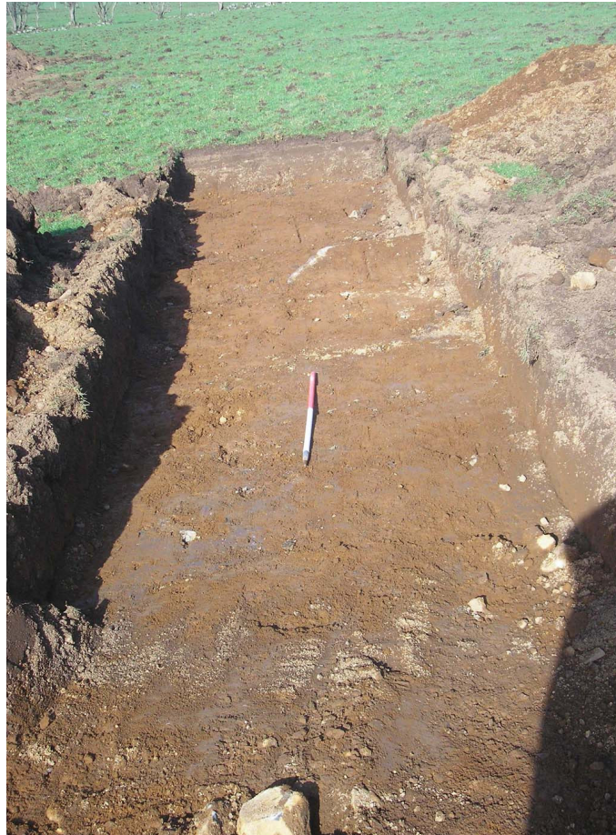
Plate 7: Trench 3 following excavation to subsoil (Context No. 303), looking north-west.
