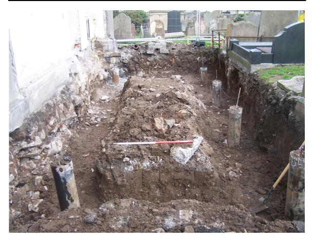
Plate 5: Evaluation area following excavation of the strip foundations around the piles, looking east.
