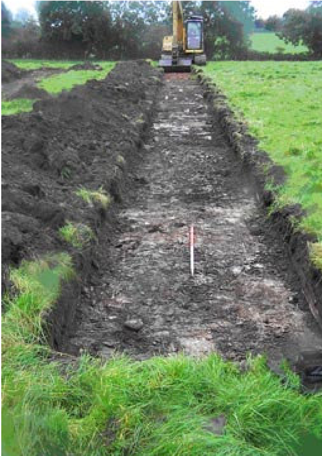
Plate 13: Trench 5 following excavation to the surface of the natural subsoil (Context No. 503). Discoloration in the subsoil is due to spoil slippage.
