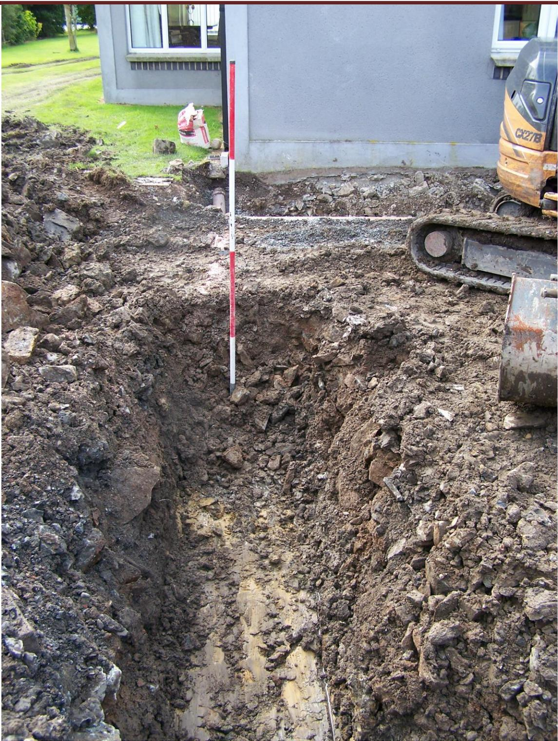
Plate 7. Subsoil clay (Horizon 6) exposed below Horizon 5, in the base of the southern foundation trench for the walls of the extension to No. 25 Kilmood Church Road. From the east.
