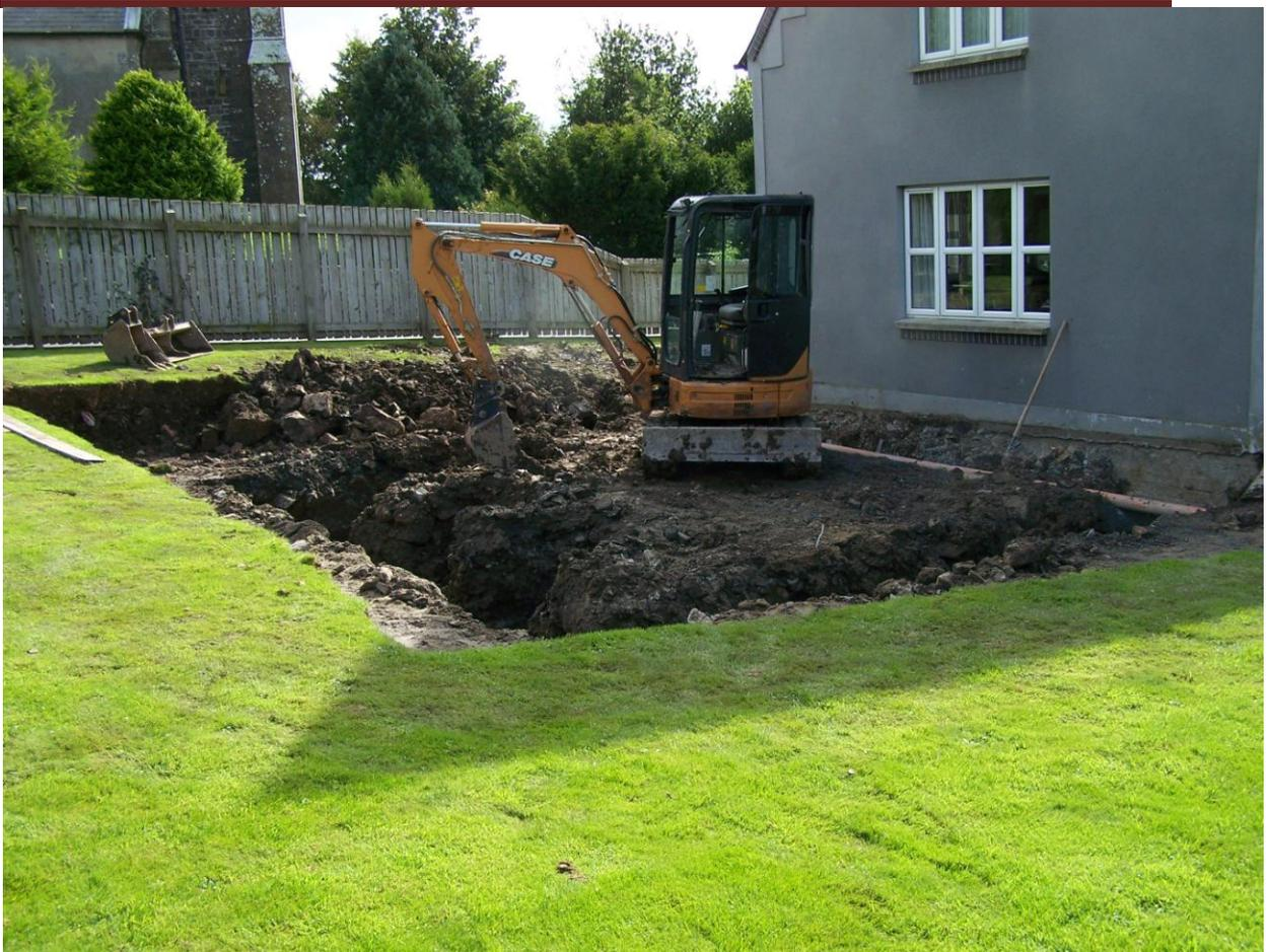
Plate 8. Completed ground works at the extension to No. 25 Kilmoor Church Road- ground reduction and wall foundation trenches. 15/09/10. From the north-east.
