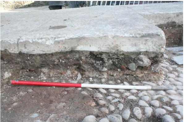
Plate 8 Concrete (C.162) overlying levelling and demolition deposits C.211 and C.209, and clay layer C.161 (over cobbles C.133) at the top of the ramp at the southern end of the Grand Battery (facing south).
