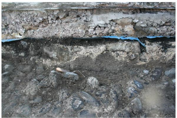
Plate 10 Surviving plaster/render on wall C.220 in Room 4; below tarp (C.105) and contemporary wall infill (C.106).
