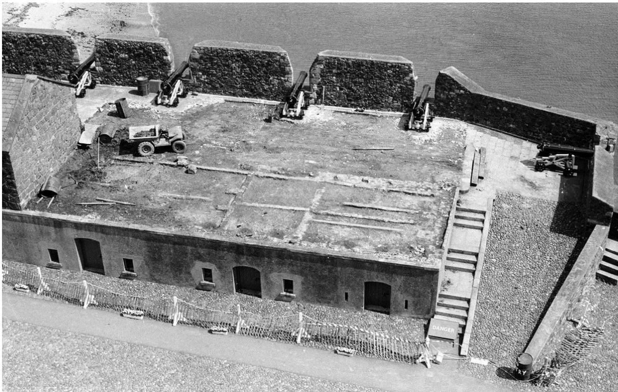
**Plate 4** The surface of the Grand Battery in 1990 when the garden was removed and the southern end was re-laid in concrete (ANT052:059-738. NIEA).
