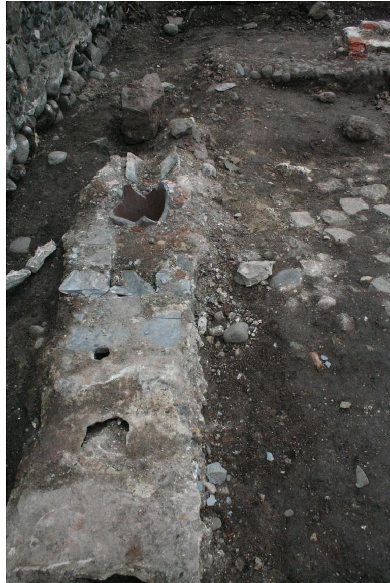
**Plate 26** Slate-capped drain (C.143), ceramic pipe (C.127) and top of Vault 5 (facing south).
