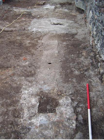
**Plate 25** Drain C.143 and integrated vent/access point with concrete pier (C.158) and pipe [covered with a stone] in the background (facing north).
