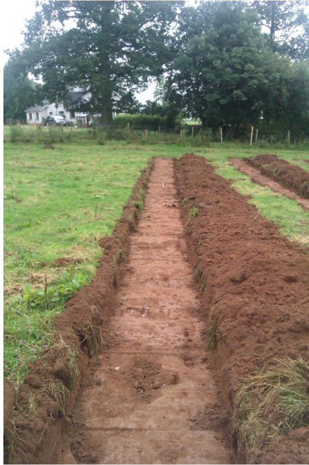
Plate 14: Trench 6 following excavation to subsoil level, looking south
