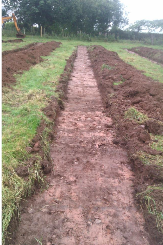
Plate 8: Trench 3 following excavation to subsoil level, looking south
