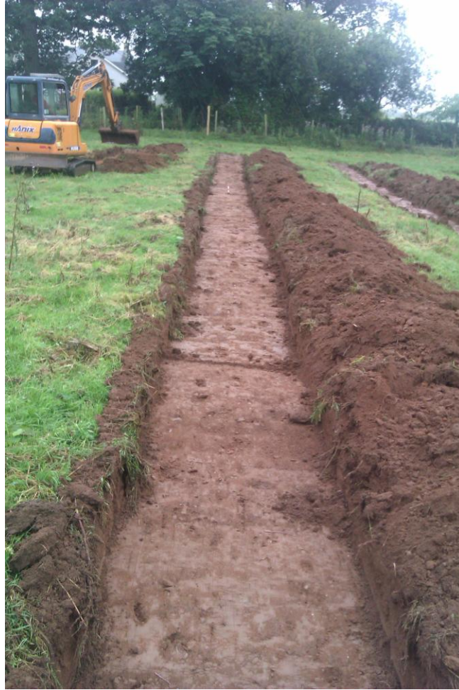
Plate 10: Trench 4 following excavation to subsoil level, looking south
