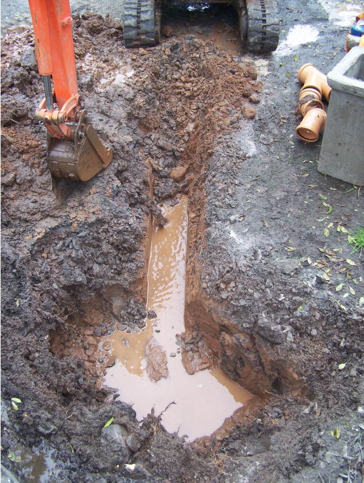
Photo 1: Excavation trench showing cut for grating and drainage gully showing orange brown clay subsoil beneath tarmac and gravel road surface
