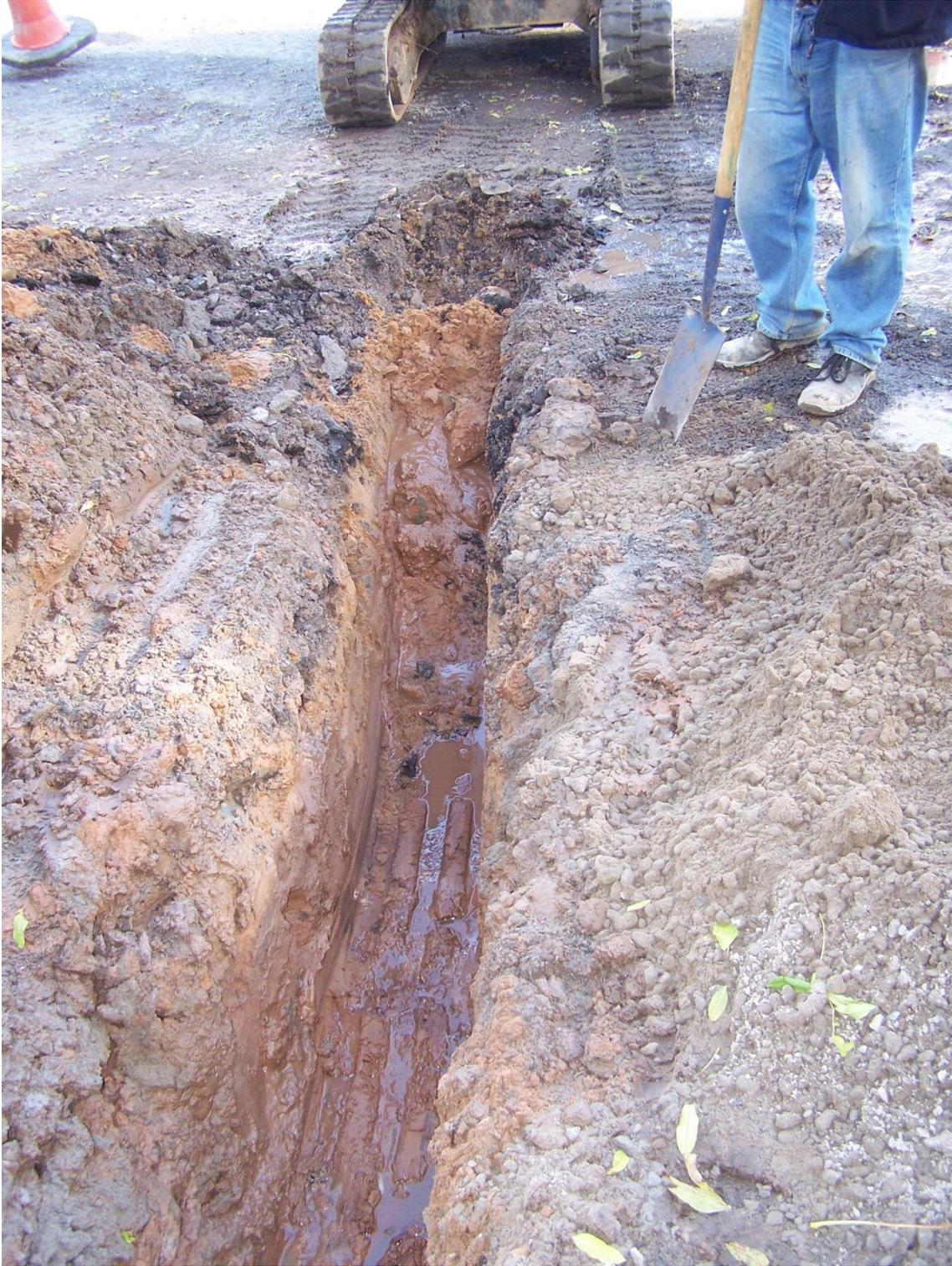
Photo 2: Continuation of cut for drain
