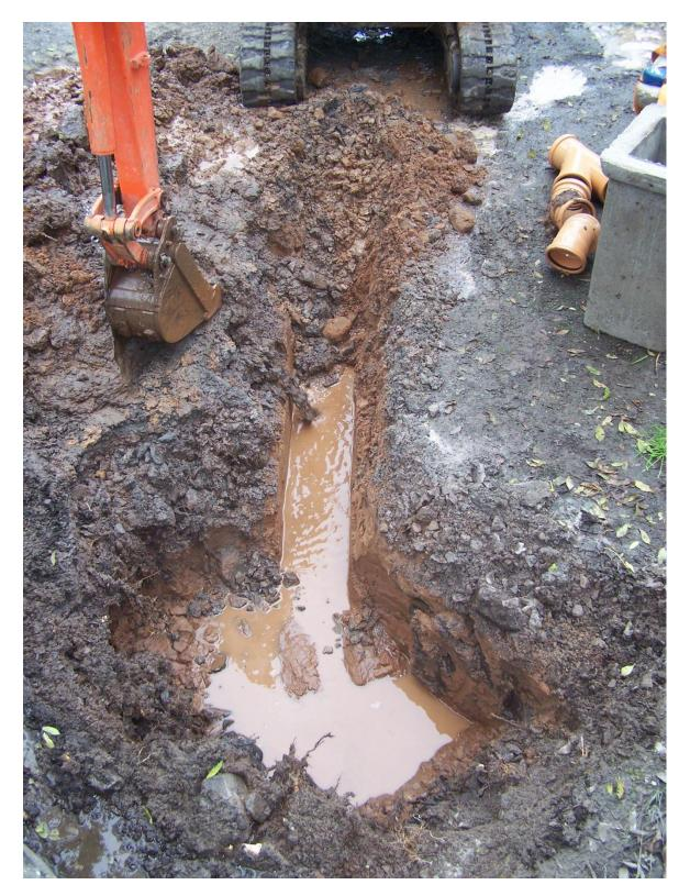
Photo 1: Excavation trench showing cut for grating and drainage gully showing orange brown clay subsoil beneath tarmac and gravel road surface
