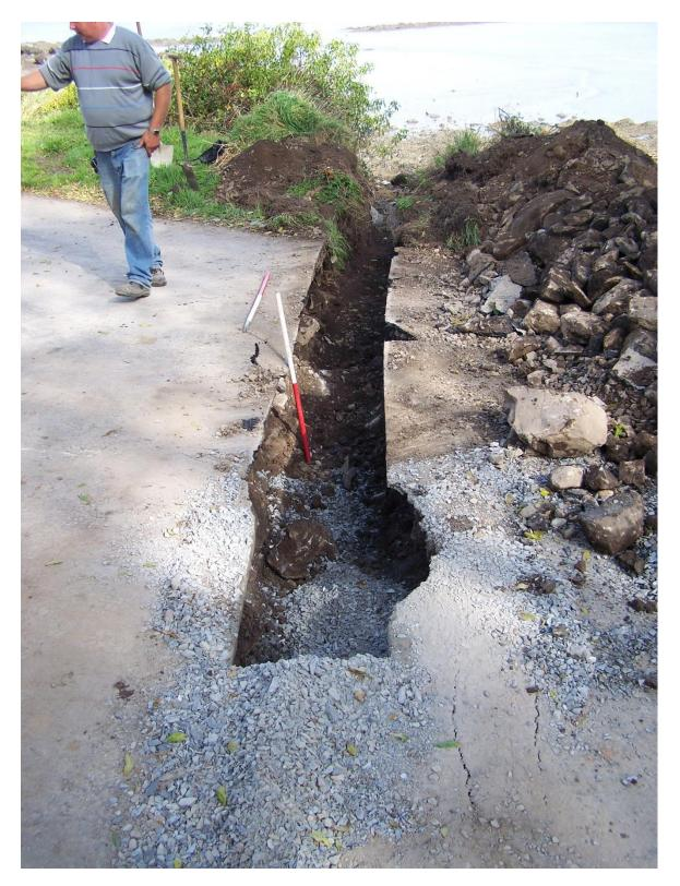
Photo 4: Final section of cut for drain extending to shoreline
