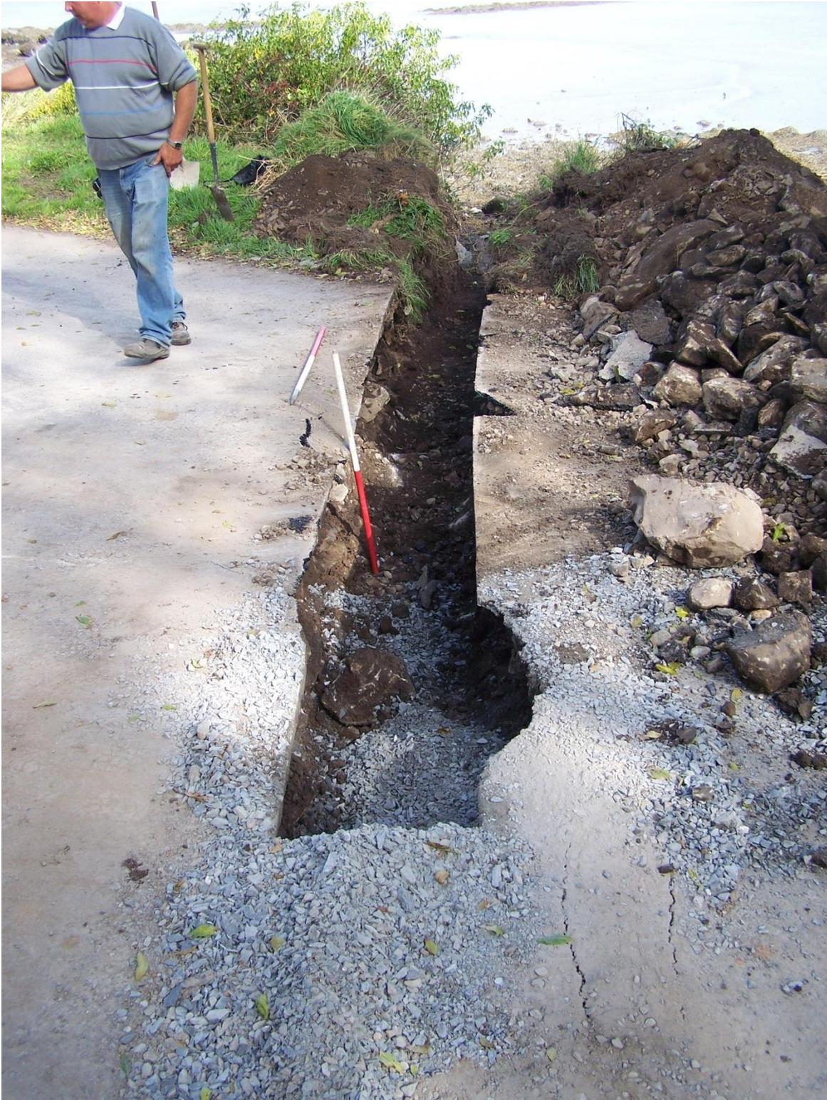
Photo 4: Final section of cut for drain extending to shoreline
