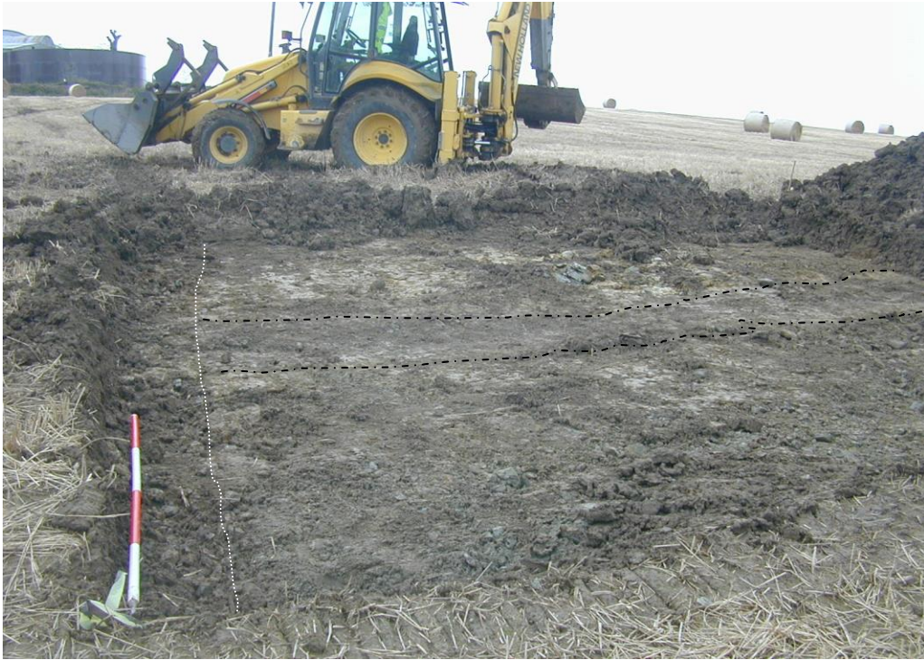
Plate 1 Mechanically excavated trench (7m x 7m) centred on the Viking silver find-spot location – photo shows the ploughsoil, subsoil and field drains (facing north).
