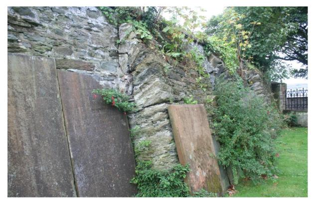
**Plate 3** The buttressed north facing wall of St Augustine's graveyard. The buttresses are not keyed-in and are clearly secondary. The excavation trench is located on the other side of the wall.
