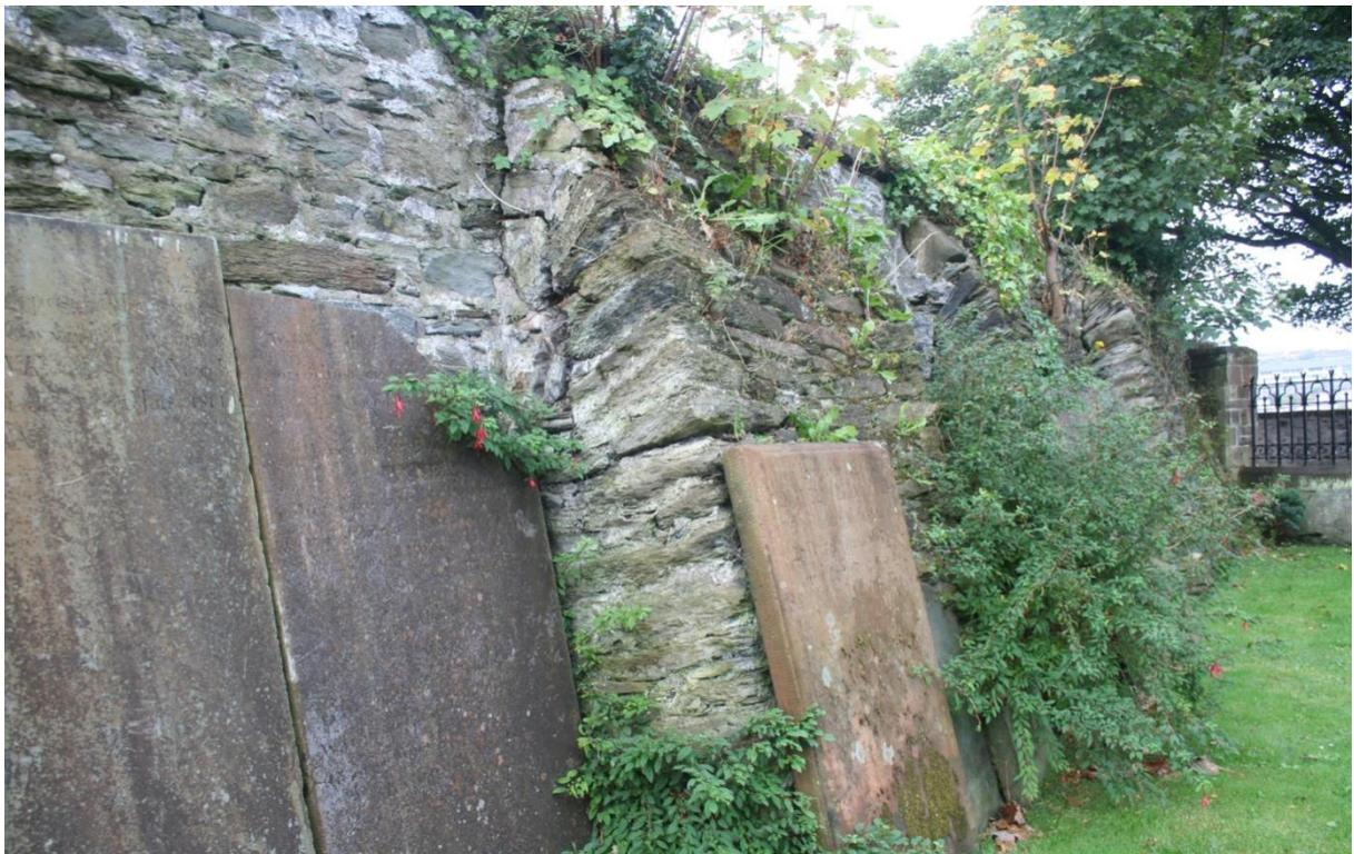
**Plate 3** The buttressed north facing wall of St Augustine's graveyard. The buttresses are not keyed-in and are clearly secondary. The excavation trench is located on the other side of the wall.
