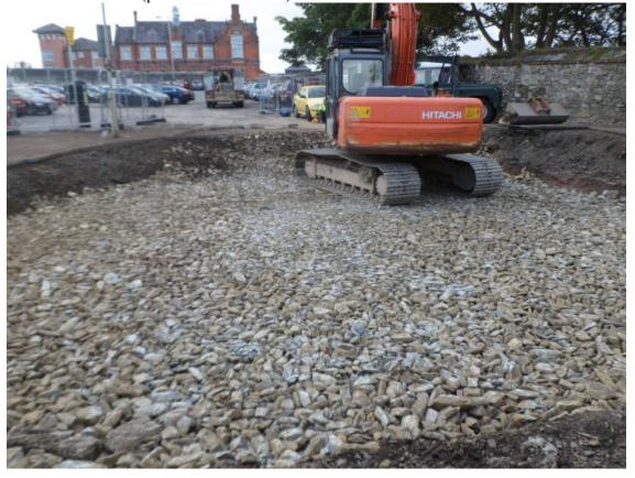
Plate 52 Backfilling of the trench.
