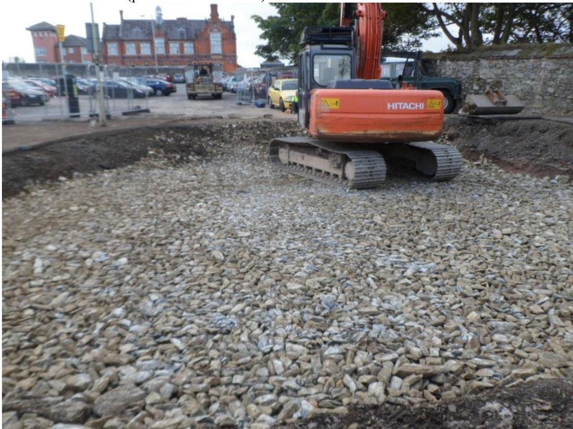
**Plate 52** Backfilling of the trench.
