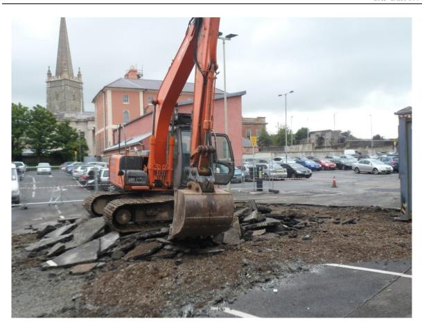
Plate 5 Removal of the tarmac C.1001, showing the hardcore, C.1002, underneath.
