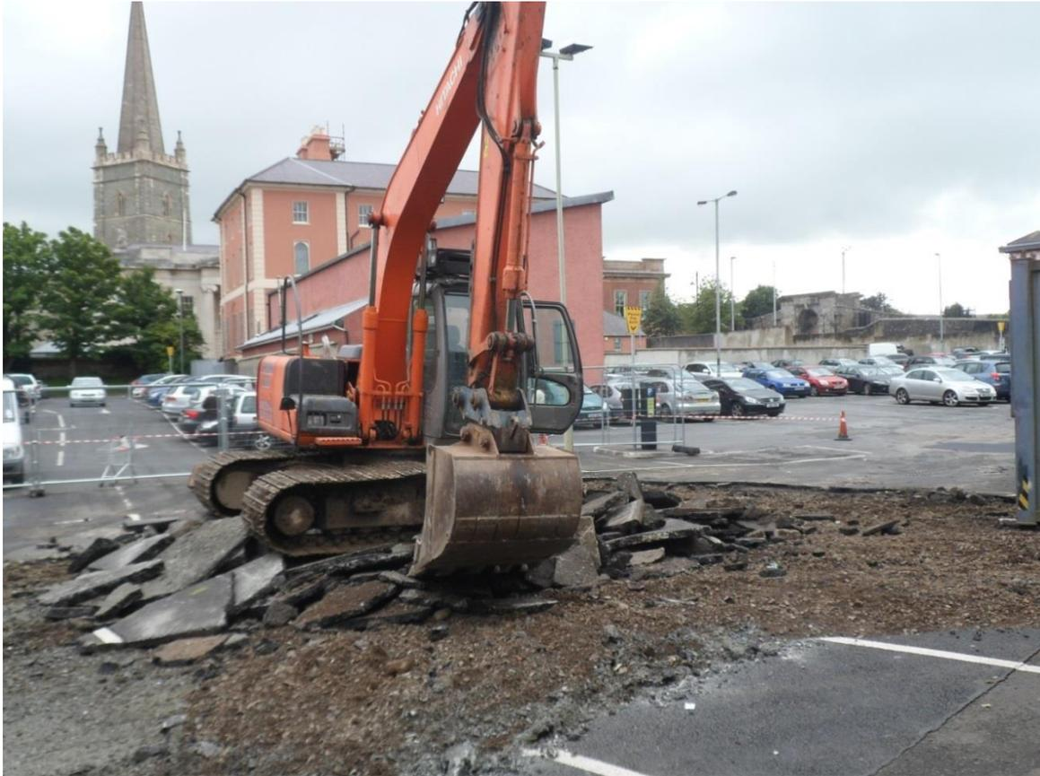
**Plate 5** Removal of the tarmac C.1001, showing the hardcore, C.1002, underneath.
