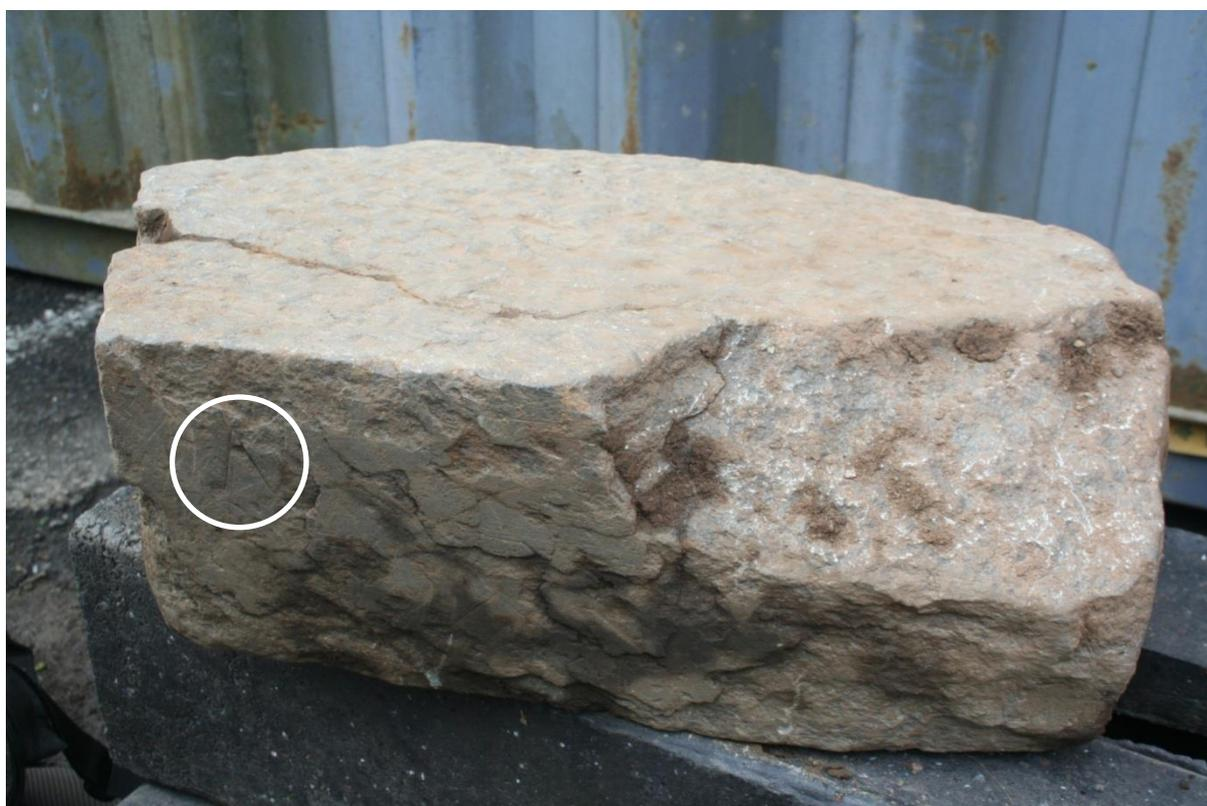
**Plate 35** View of the cut and dressed stone after it was lifted showing scratches and possible mason's mark 'A' (circled).
