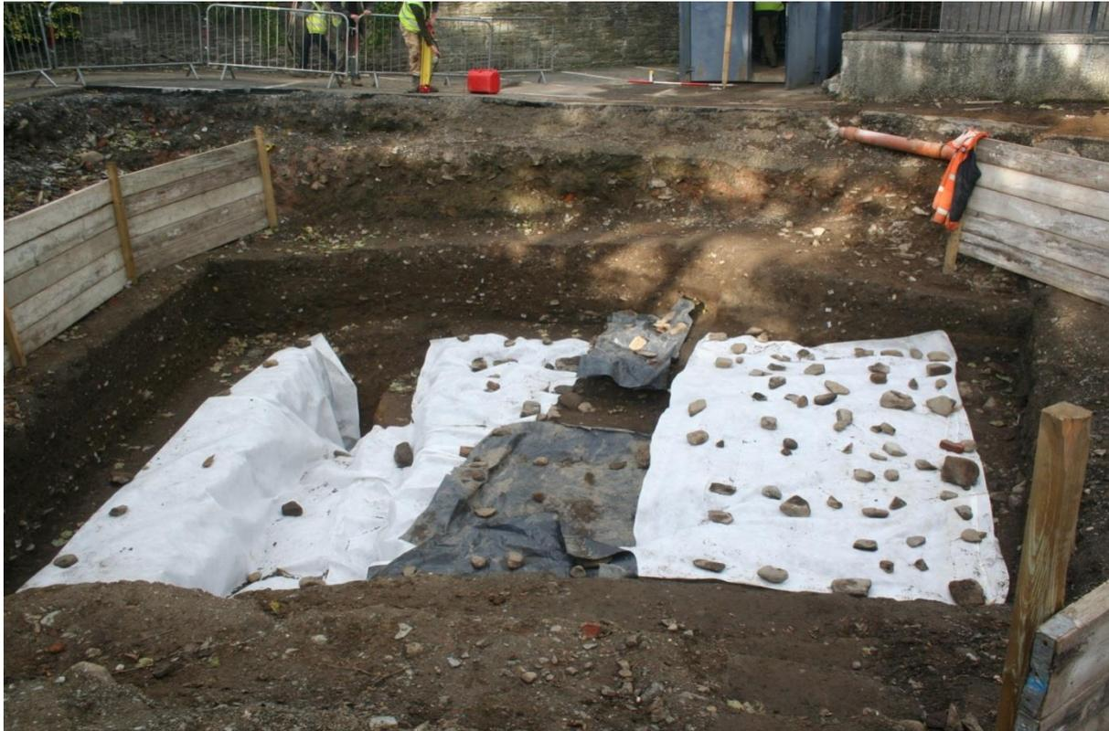
**Plate 51** The terram (permeable membrane) laid down over the base of the trench before it was back-filled.
