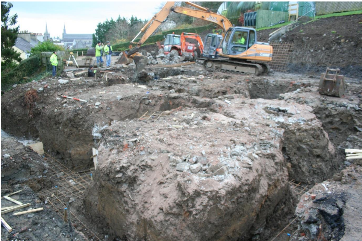
Plate 2 – Site following excavation of foundations (looking south east)
