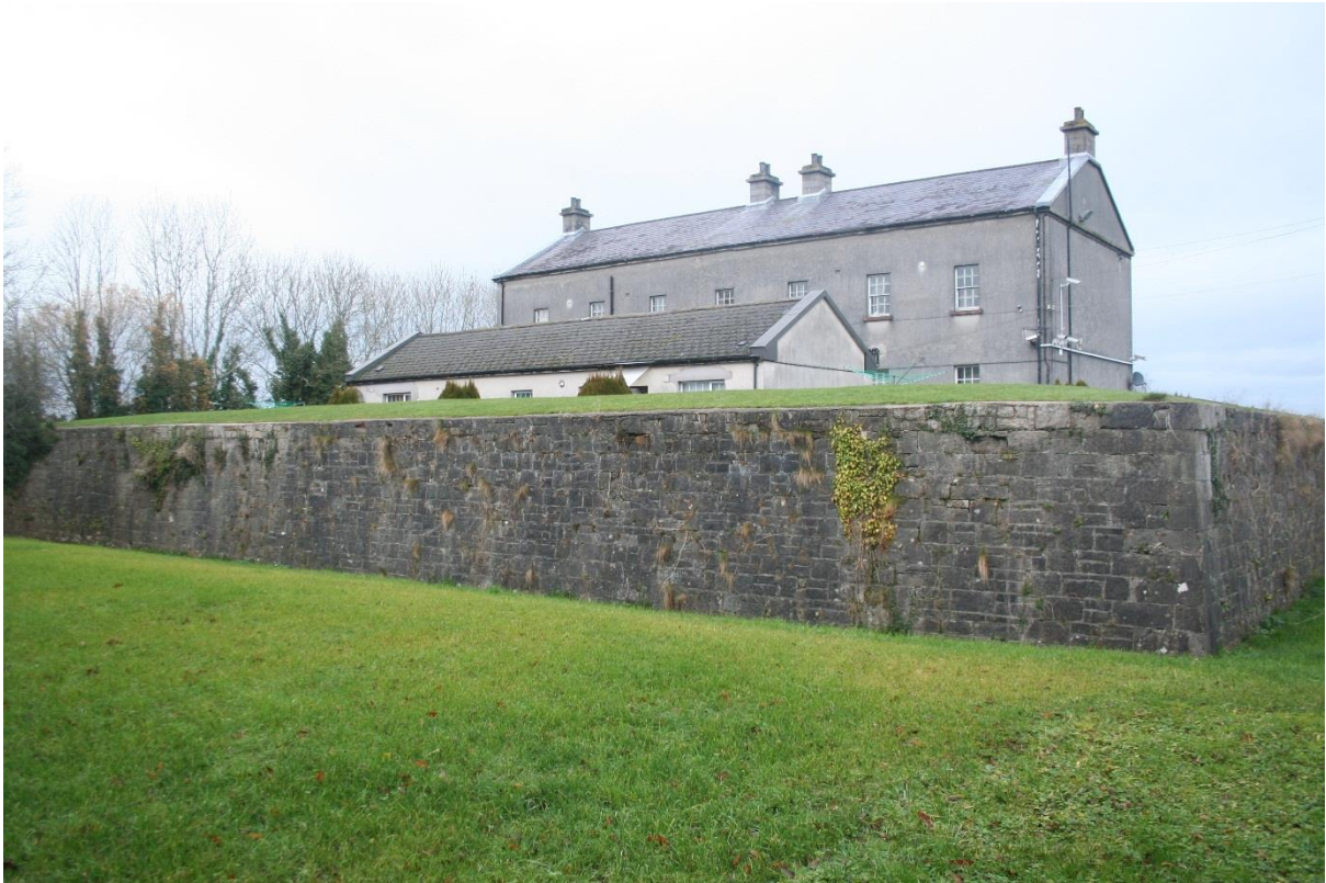
Plate 1 – The Redoubt, West Fort (looking north west)
