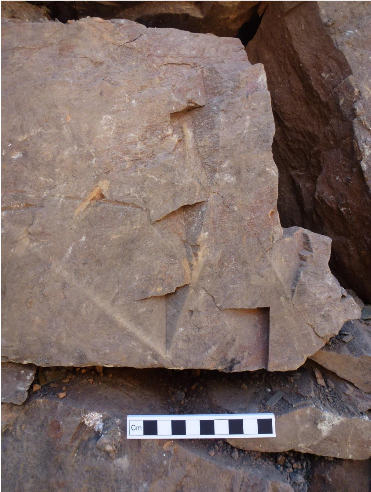
Figure 30: Apparent tool marks within the fabric of the internal, faced wall of the lime kiln (511).
