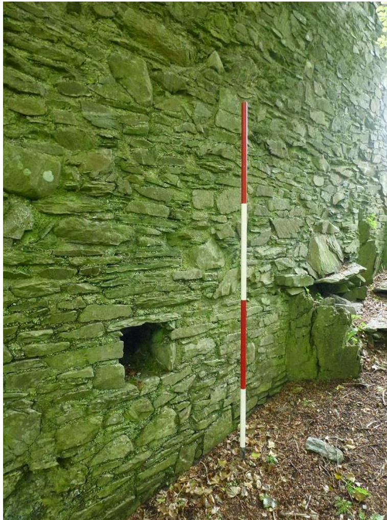
Figure 9: Probable latrine chute in the external face of the northeastern section of the outer ward's curtain wall, looking west.
