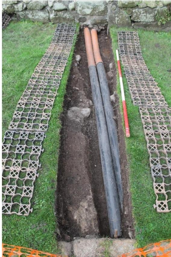
**Plate 12. Trench 11. Shot of southern end of the trench showing the modern plastic pipes (C1103/ C. 1108 and C. 1104/ C. 1007) within their foundation trench (C. 1109) running through the Middle Ward curtain wall (C. 1114). Looking south.**
