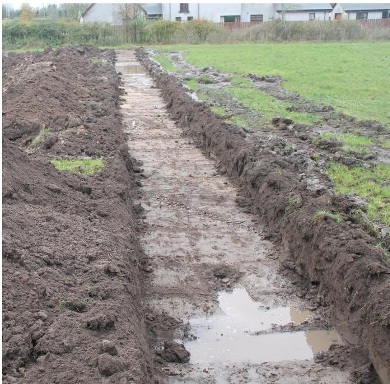
Plate 15. Ardboe, Co. Tyrone. Looking back along Long Trench 8. Stone drain with red brick cut into subsoil in foreground, two field drains running diagonally across the trench in the middle of the shot and water covering a field drain at the eastern end of the trench in the background. From the east.
