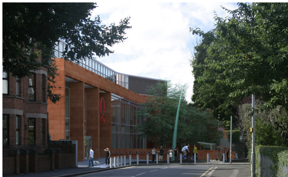
New Building Main Entrance on Chlorine Gardens, viewed from Stranmillis Road
