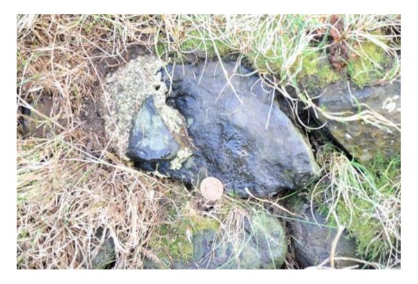
Figure 11 (DSC 1820): Mortar bonding on inner face of northern wall
