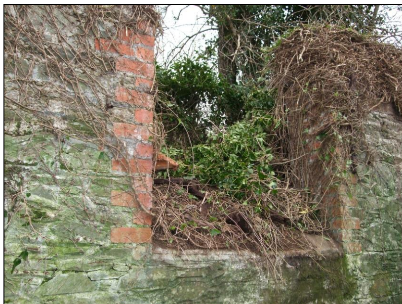
Fig. 32: Interior of Coal Store: chute (3.3.3). (DSCF0840)
