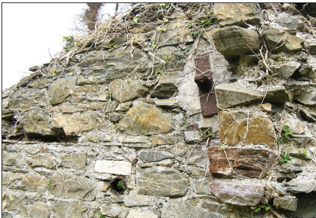
Fig. 39: Interior north wall of purifier house: through-pipe and iron bracket. (RIMG0113)
