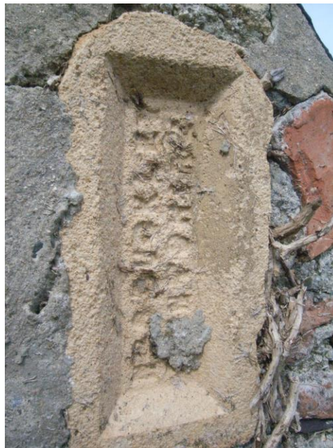
Fig. 34: Buckley brick in merlon. (RIMG0109)
