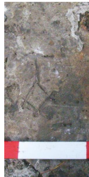
Fig.19 Mason's mark (RIMG0076)
