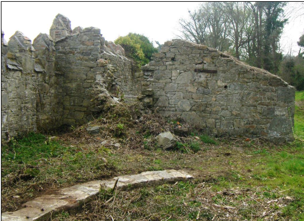
Fig. 38: North wall of gashouse, exterior. (RIMG0021)
