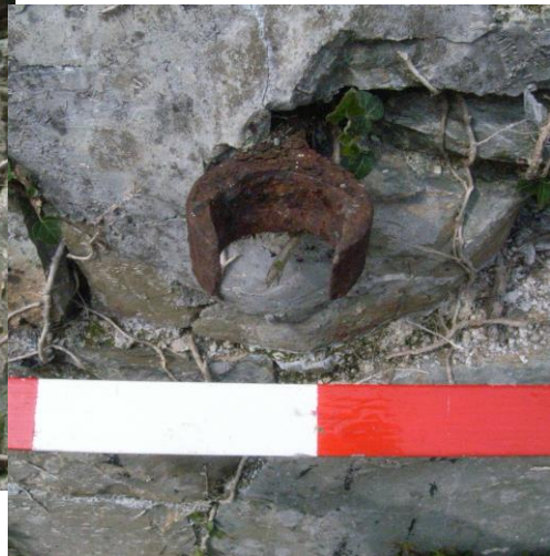
Fig. 45: Purifier house. (RIMG0118)
