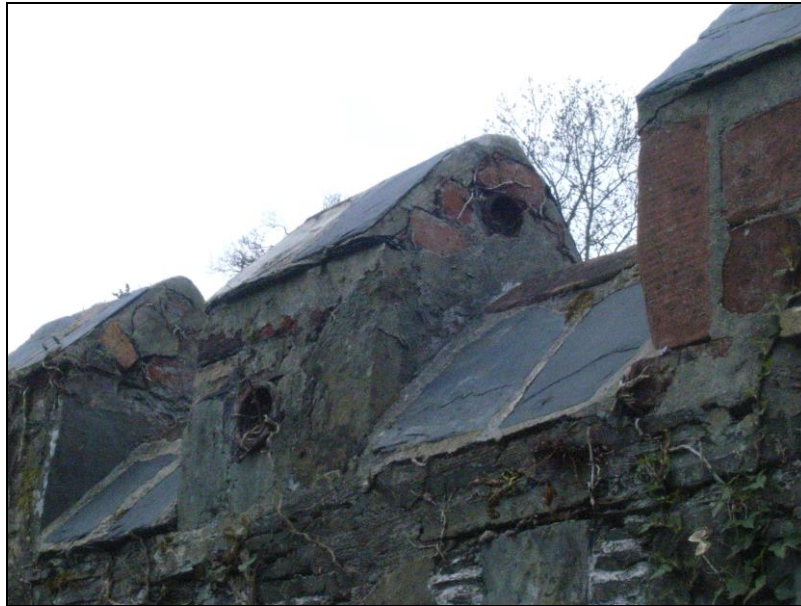
Fig. 23: Merlon near gasholder. (RIMG0092)
