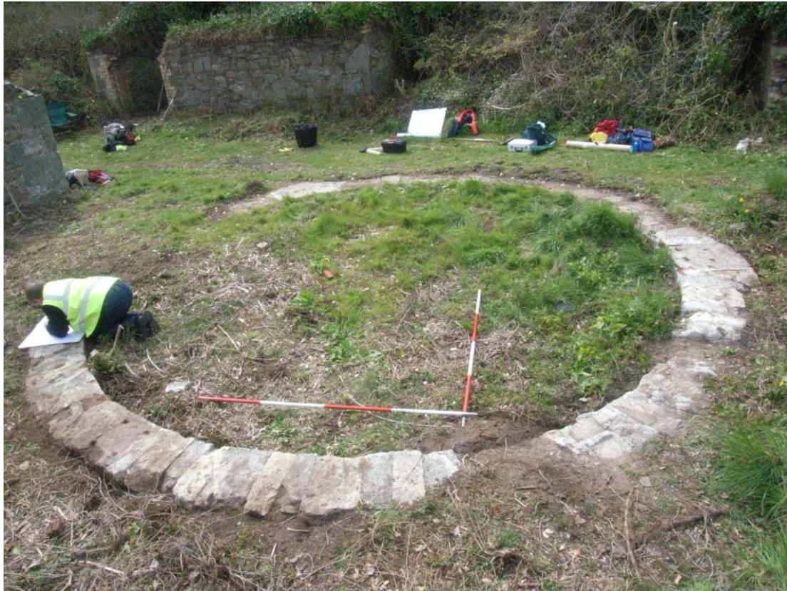
Fig. 17: Coping of gasholder tank. (RIMG0110)
