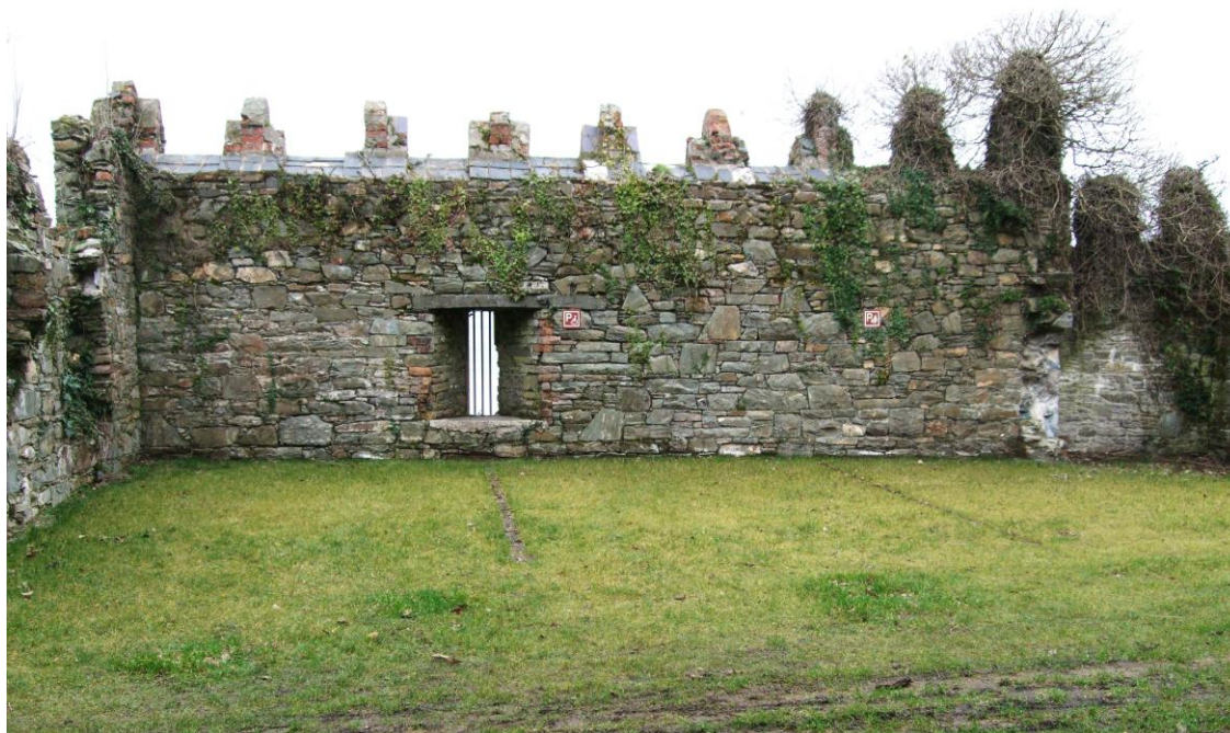
Fig. 40: The gashouse in 2012. (DSCF1443)
