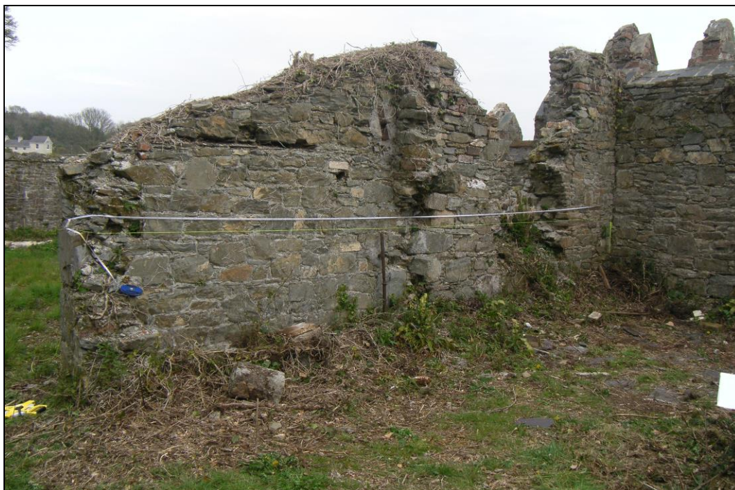
Fig. 12: North wall of Gashouse, interior. (RIMG0007).
