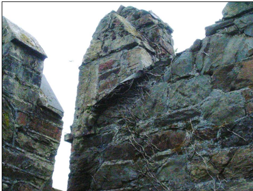
Fig. 26: Merlon at NE corner of gashouse. (RIMG0097)
