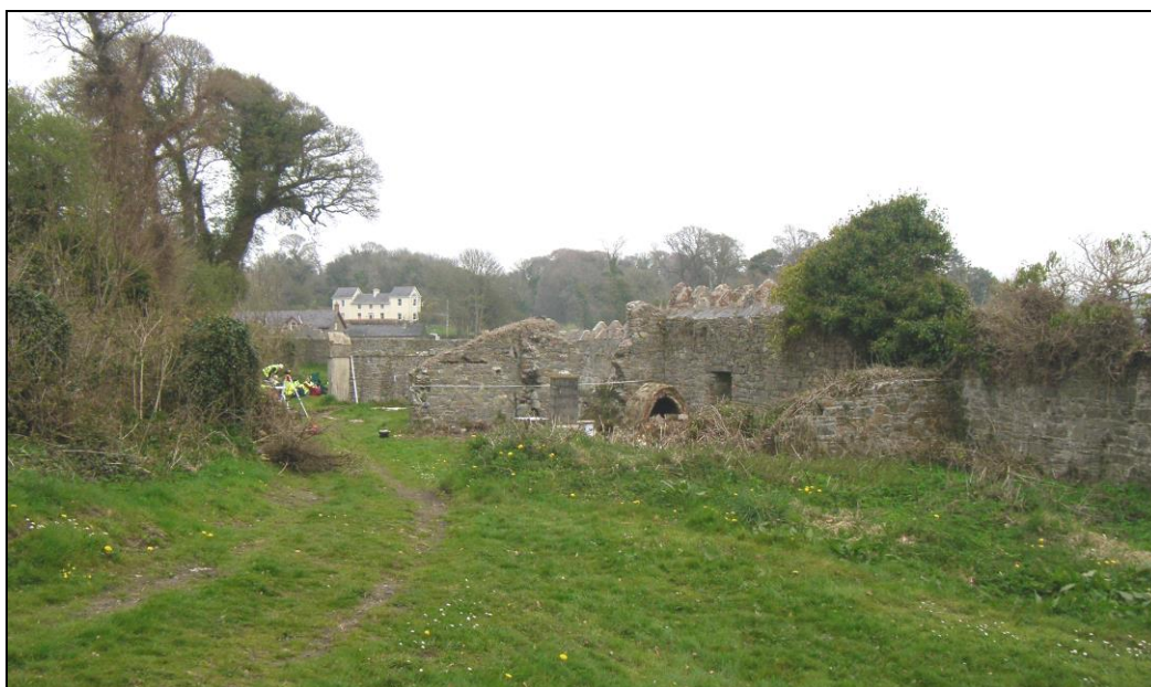
Fig. 7: General view of gasworks from SW. (RIMG0003).
