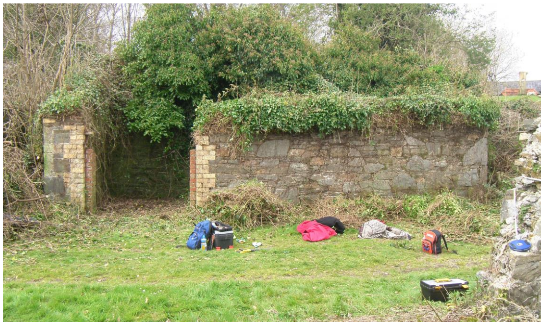
Fig. 16: Coal Store viewed from the east. (RIMG0015)
