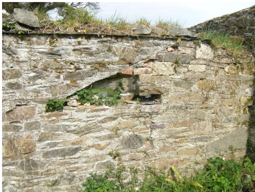
Fig. 21: North yard wall, interior. (RIMG0030)
