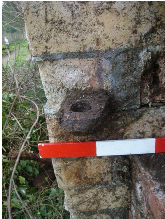
Fig. 42: Coal store door (south). (RIMG0125)
