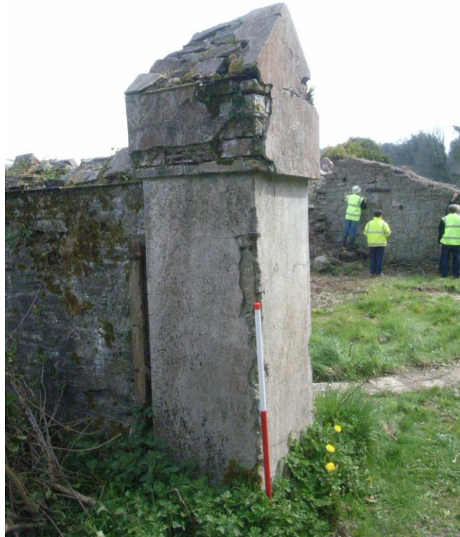
Fig. 20: North gate, east pier. (RIMG0103)
