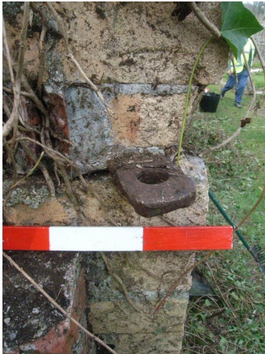
Fig. 41: Coal store door (north). (RIMG0126)
