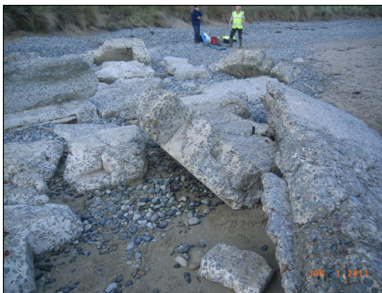
Figure 30: Angular stones set into concrete matrix
