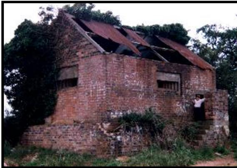
Figure 13: Large Pillbox at High Ercall, Shropshire, disguised as a house (after Matthews 2001)
