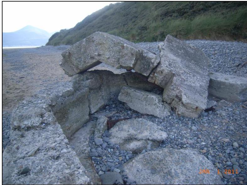
Figure 31: Iron/metal items within the Pillbox structure
