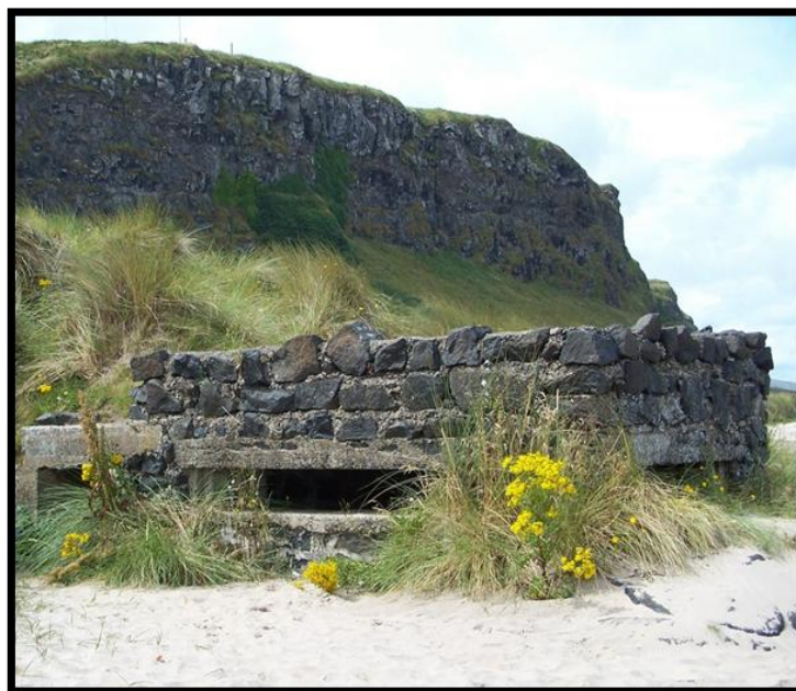
Figure 18: Downhill Pillbox, with basalt blocks as additional camouflage
