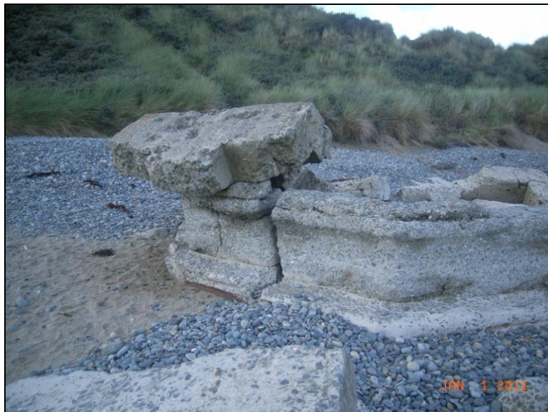
Figure 25: Elements of Pillbox still in situ
