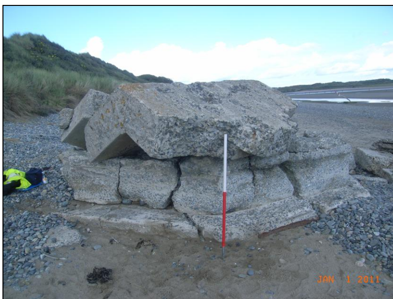
Figure 26: Evidence for sectional construction
