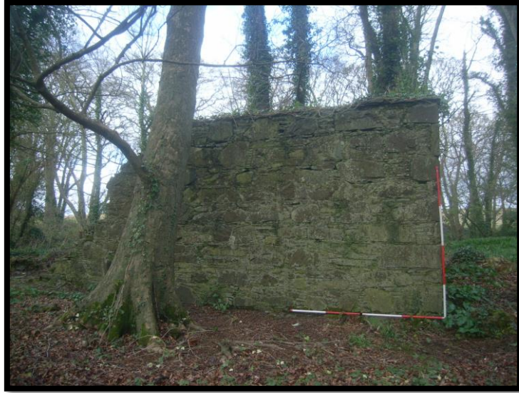
Figure 24: View of south wall, looking north
