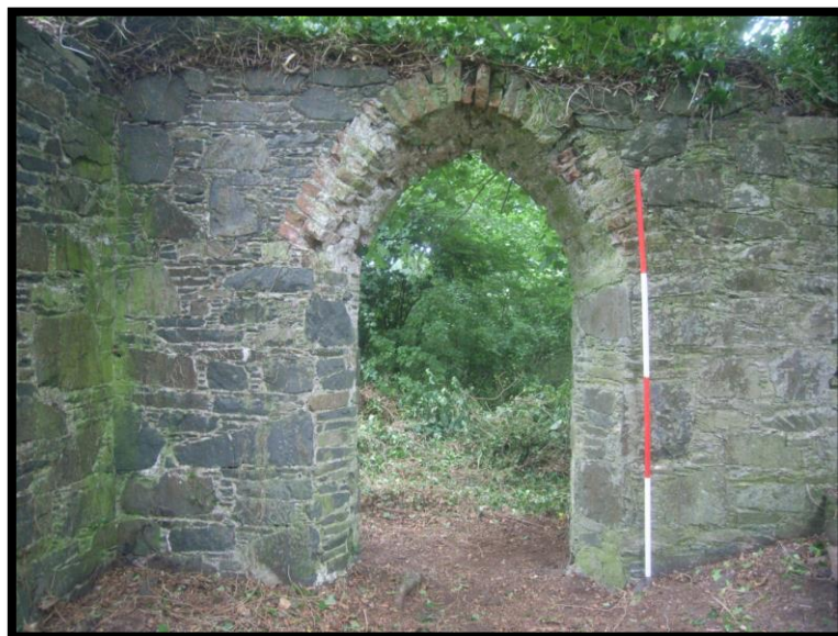
Figure 32: Doorway arch at the cottage ornée, looking north
