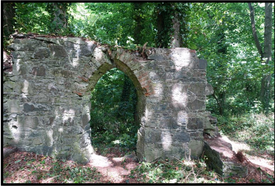
Figure 33: Window opening in north wall, looking north
