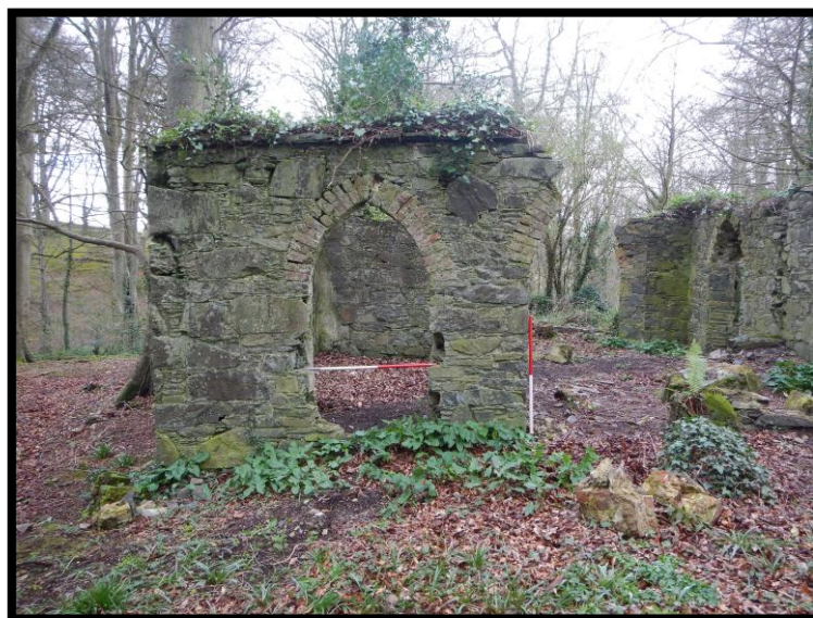
Figure 25: Window of the east wall, looking west
