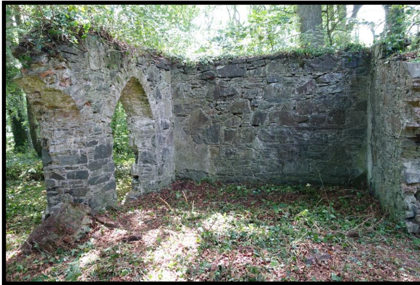
Figure 28: Internal room with window on the east wall, looking south
