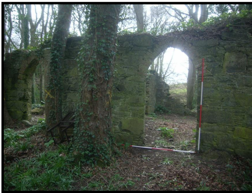
Figure 23: View of north wall, with doorway and window, looking south
