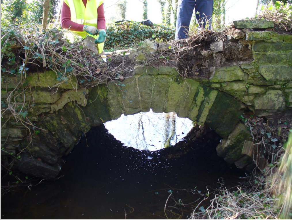
Figure 10: North-eastern face showing parapet damage
