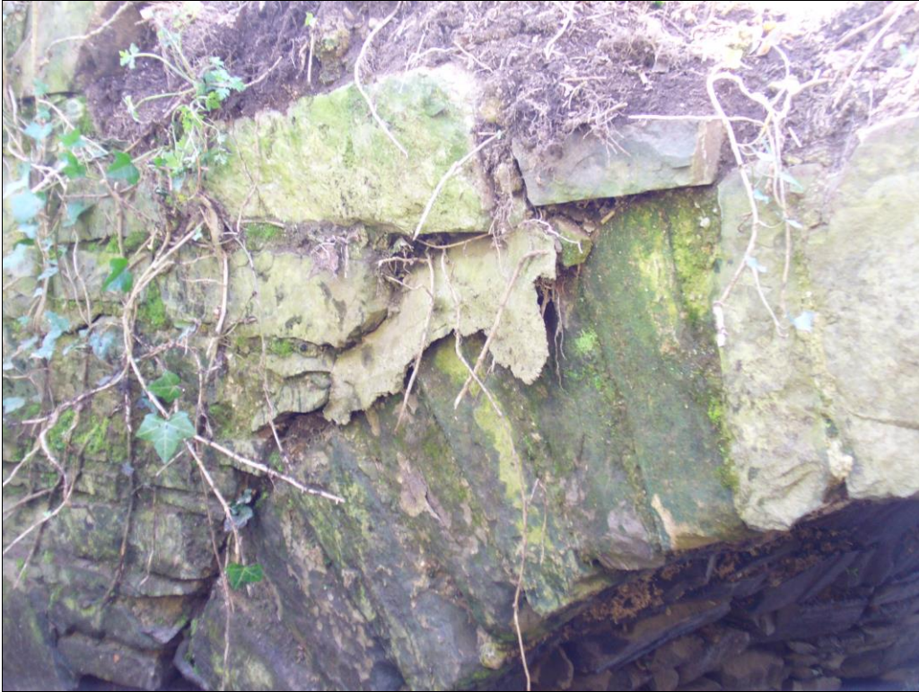
Figure 12: Detail of north-eastern face stonework
