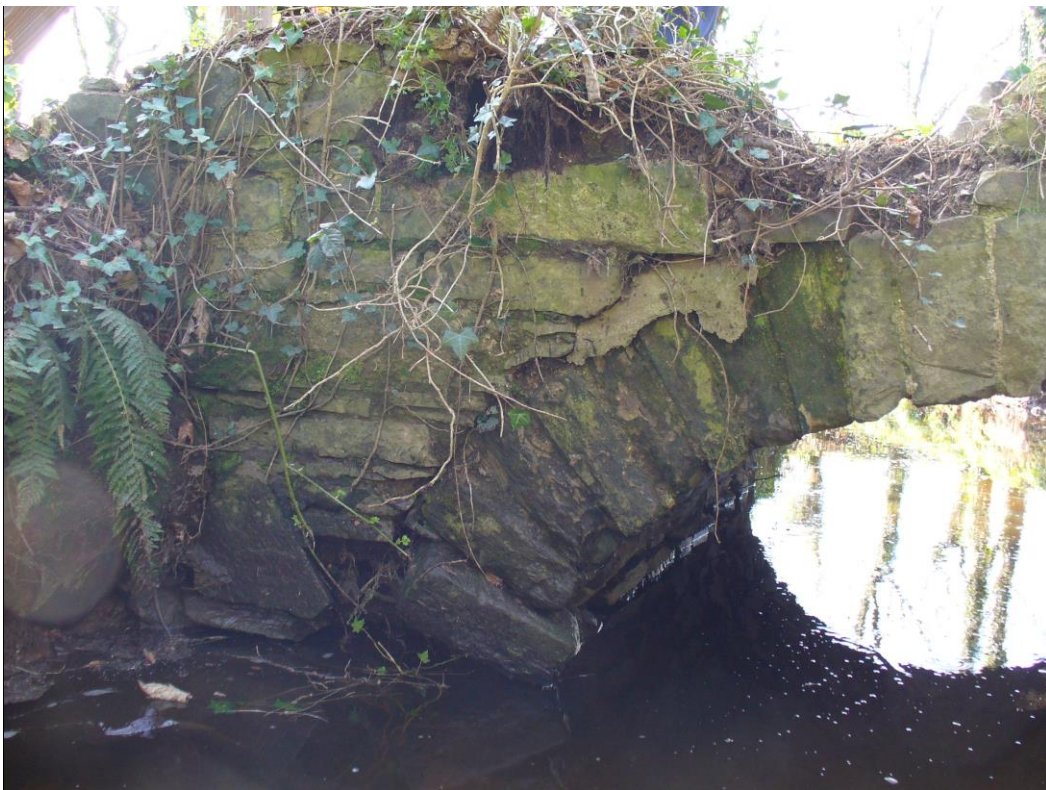
Figure 10: North-eastern face showing parapet damage
