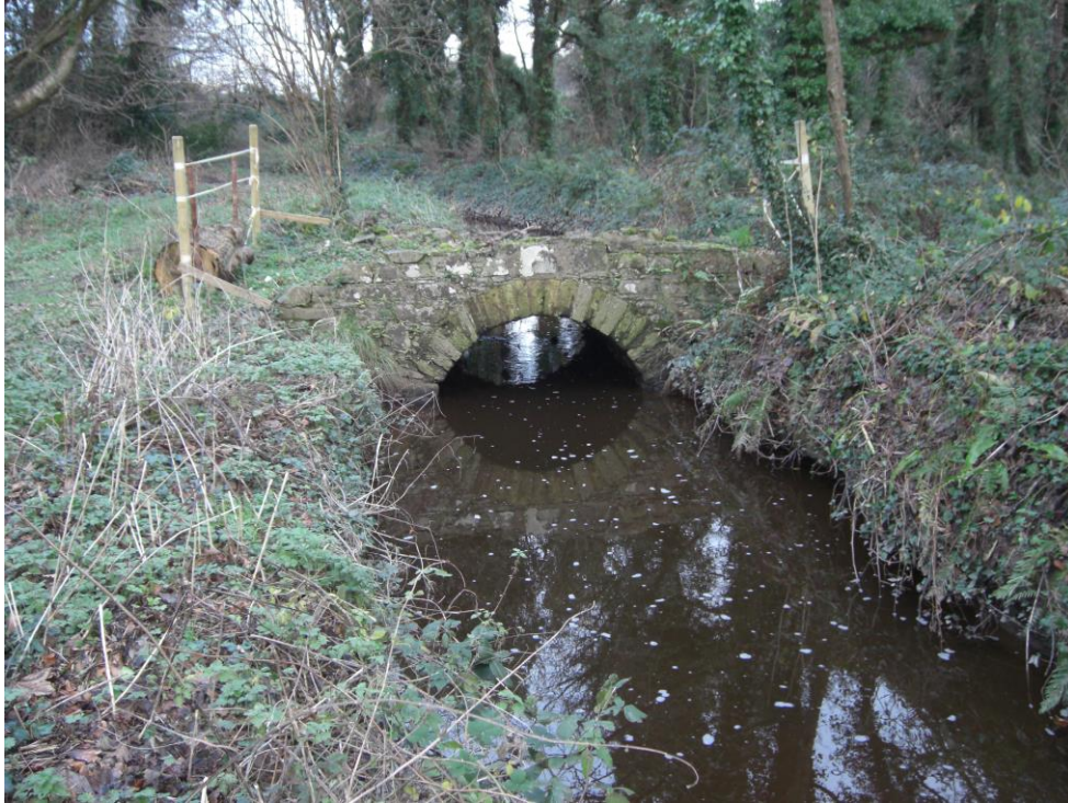
Figure 15: View of bridge with restricted access (December 2015)
