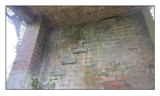
Figure 12: Showing external stairs embedded into supporting wall.
