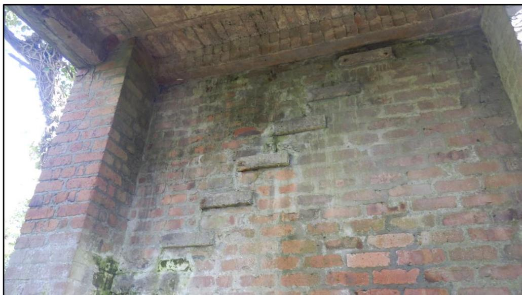
Figure 12: Showing external stairs embedded into supporting wall.
