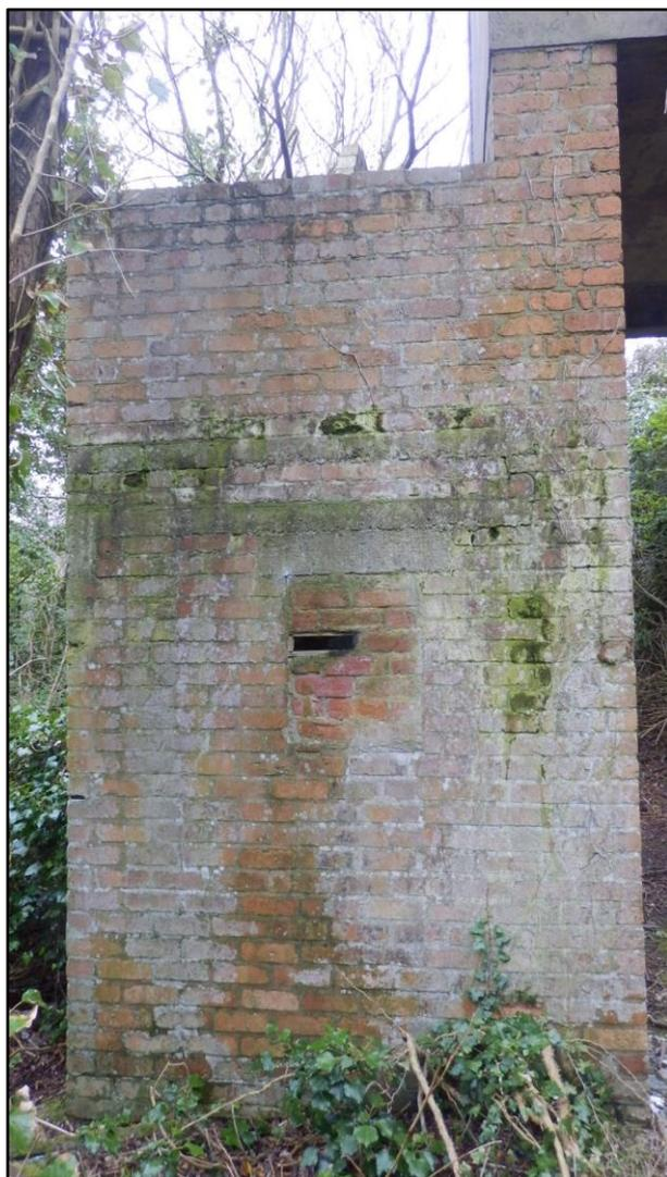
Figure 11: Part of lower north wall with widow bricked in, but a 'letterbox' aperture constructed and meshed over.
