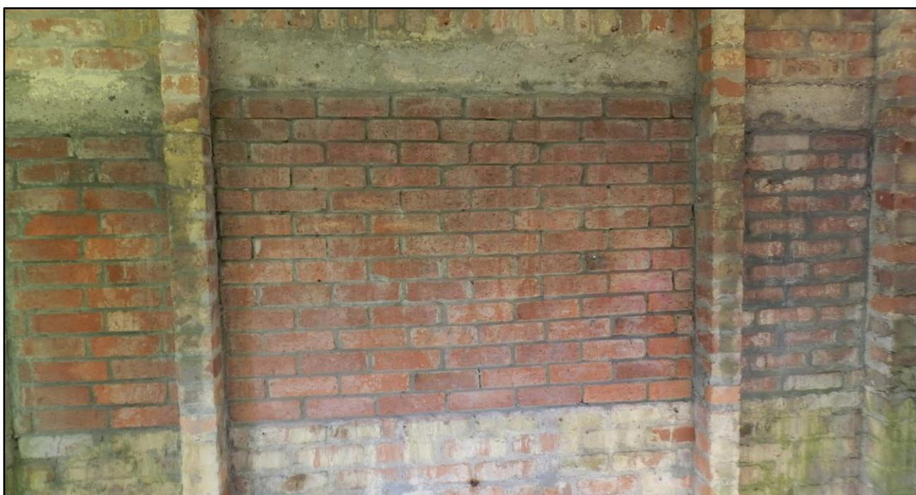
Figure 10: Interior of west wall showing bricked-up main observation windows.
