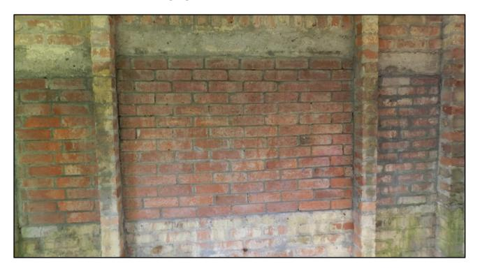
Figure 10: Interior of west wall showing bricked-up main observation windows.
