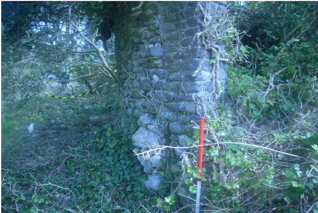
Figure 40: Lower wall tied into terrace.
