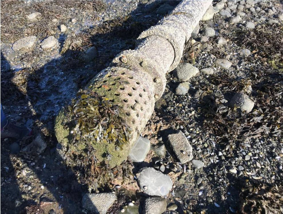
Figure 55: View of seawater intake pipe for pool, taken in October 2018. Note the supports have deteriorated and no longer support the final section of the pipe.
