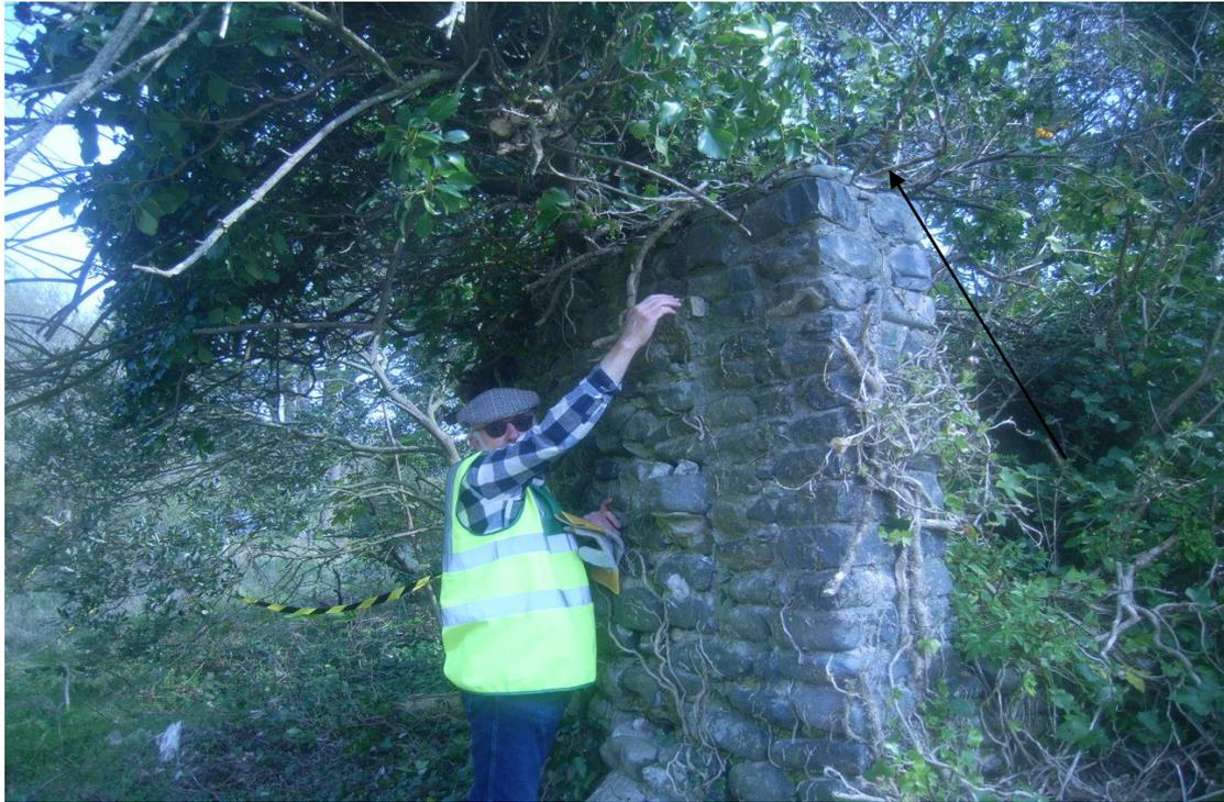
Figure 41: Upper wall tied into terrace structure
