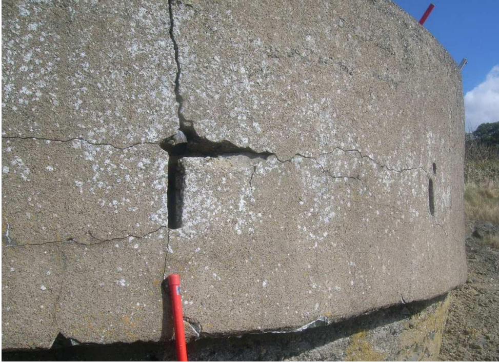
Figure 15: Vertical and horizontal cracks. The horizontal cracks follow the junction of the protective wall and the platform, looking east
