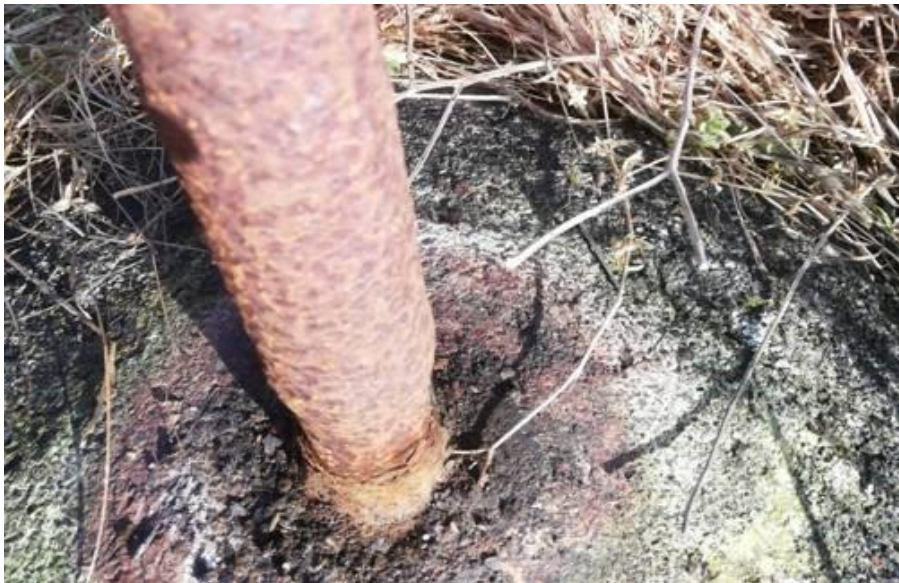
Figure 12: Close-up of the base of the axle showing corrosion
