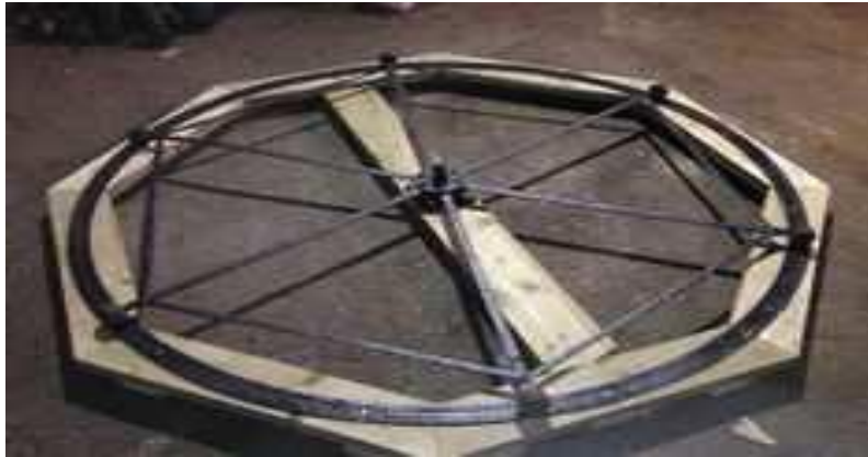
Figure 09: The chassis of a modern revolving summer house on which the wooden structure would be built. The original Mount Stewart one would have been very similar.
