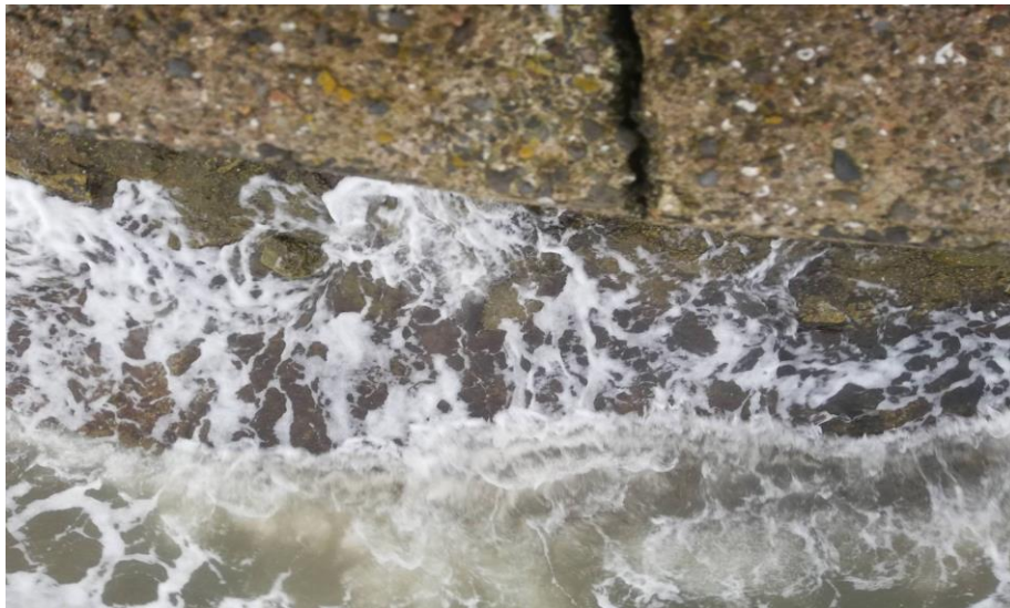
Figure 22: Waves undermining the base on a typical tide.
