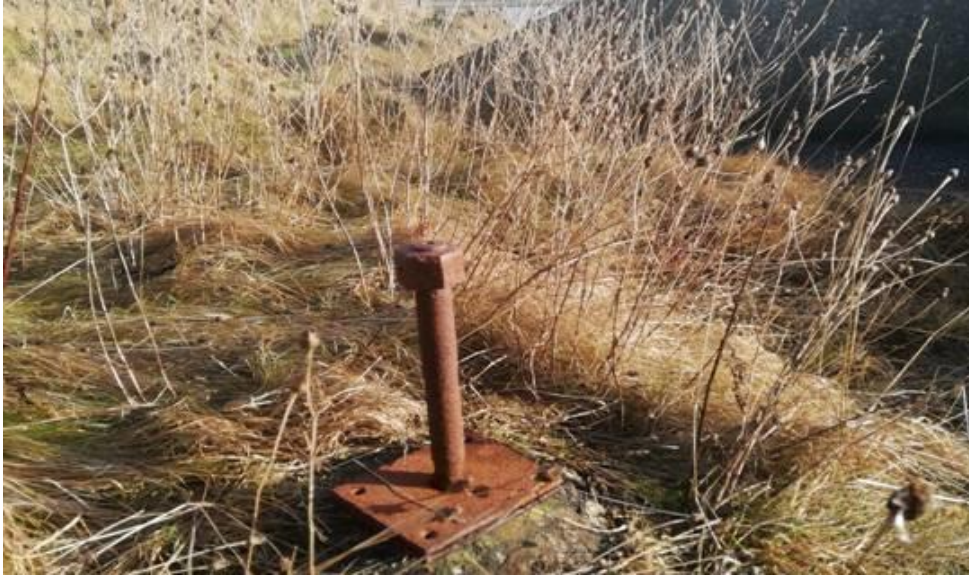
Figure 11: View of the central iron axle with a mounting plate
