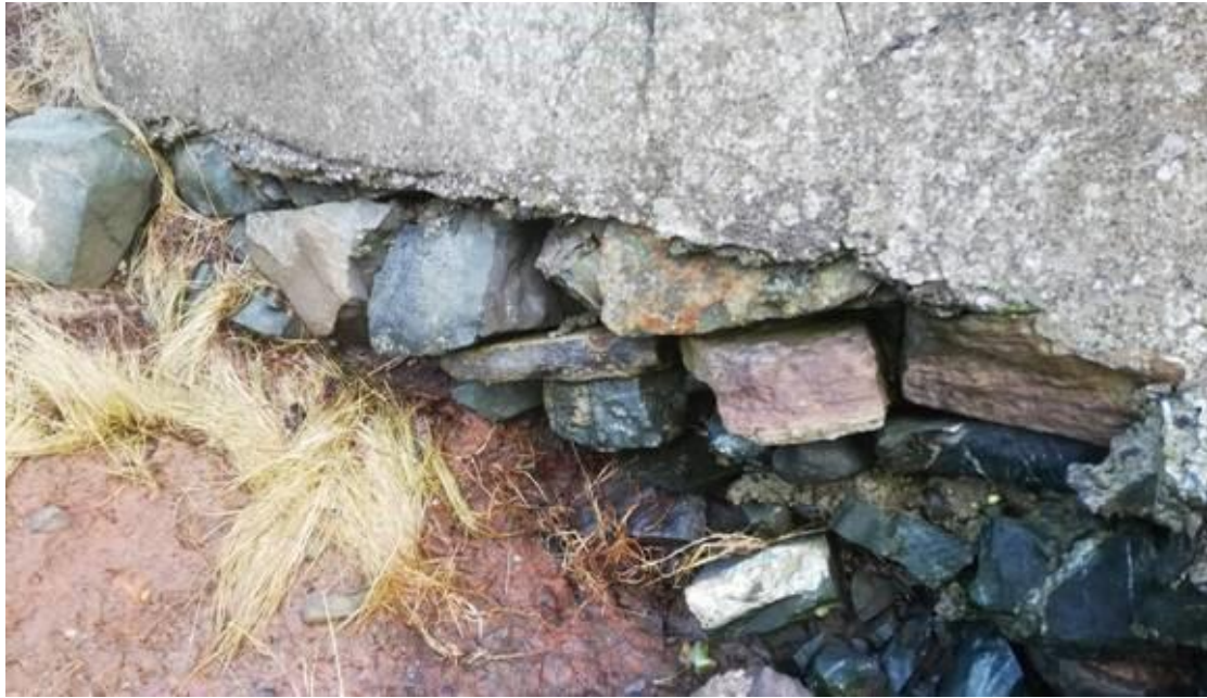
Figure 19: View of poorly-mortared matrix
