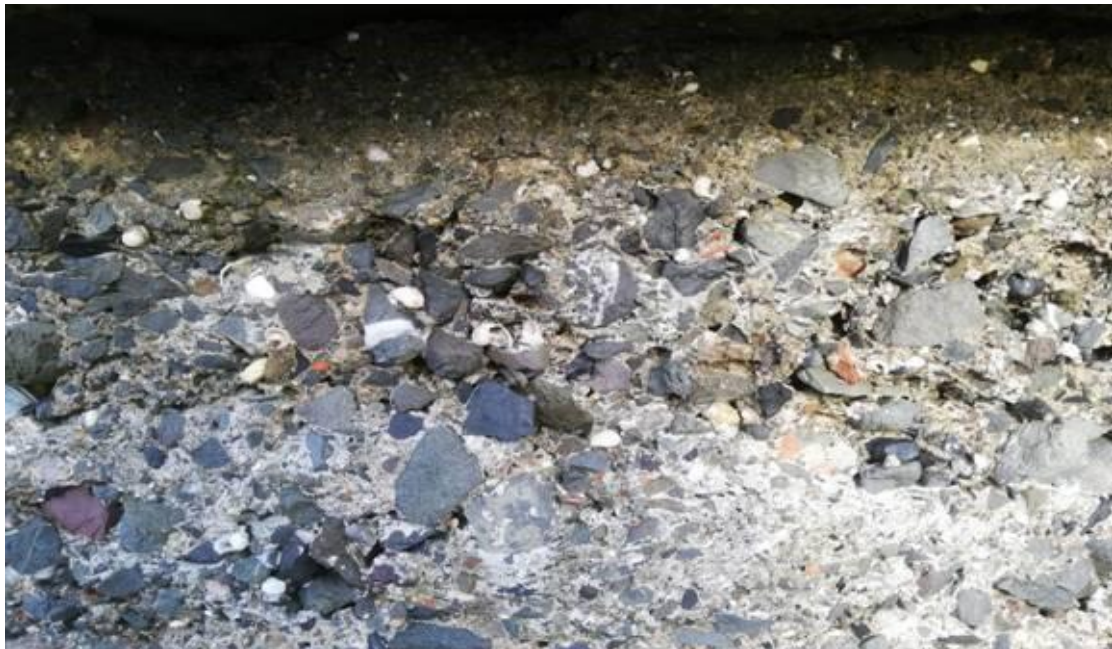
Figure 20: View of intermediate concrete mix
