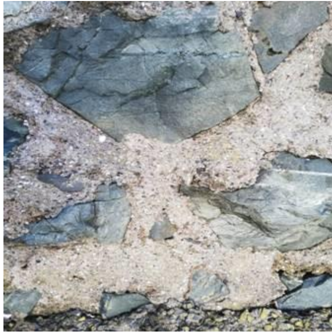
Figure 21: View of base concrete mix, with larger stone matrix
