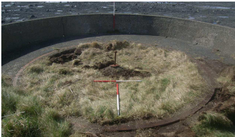
Figure 10; The Mount Stewart summer house protective wall, circular platform, iron rail and central axle, looking west.
