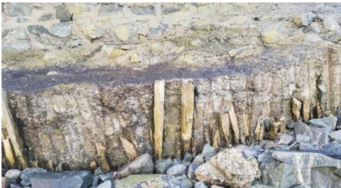
Figure 18: Remains of wooden shuttering at the base
