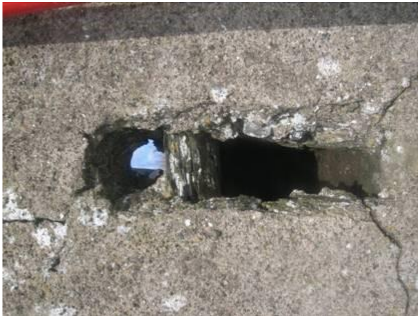
Figure 14: Hole in the wall showing cracks going right through the wall.
