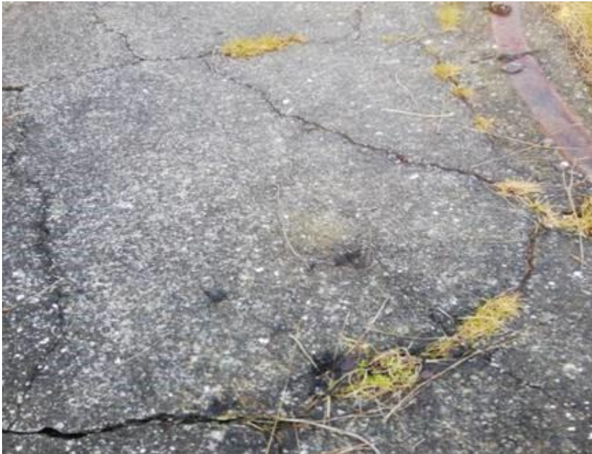
Figure 16: Cracks on the concrete circular platform for the sun house near the iron rail
