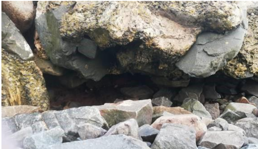
Figure 24: Undermining of the base of second summer house
