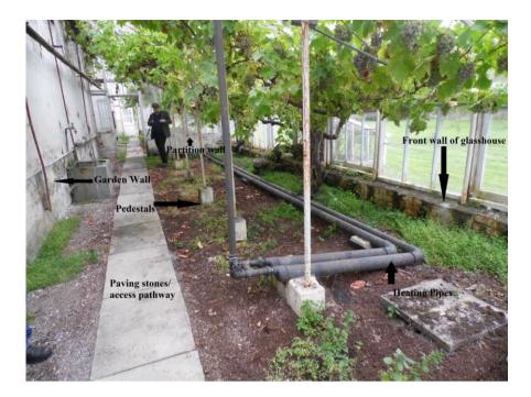
Figure 16: View of surviving internal arrangements of a vinery glasshouse located within the Walled Garden at Mount Stewart in County Down *M. Conway*
