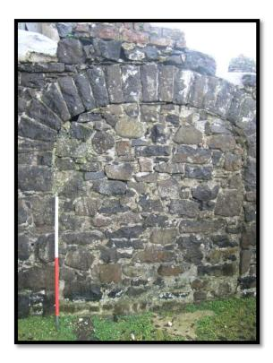
Figure 22: Blocked-up arch in the south wall of Room 1, looking south
