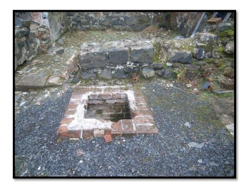
Figure 31: Inspection hatch to main drain situated outside Room 3 in the East Yard, looking east
