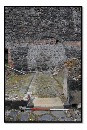
Figure 21: Evidence for large blocked-up arch, precise stone kerbing and cobbles, looking east
