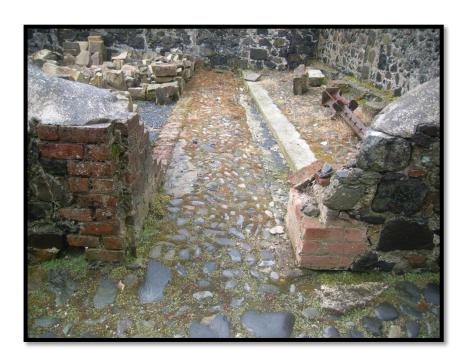
Figure 10: Original cobbled surfaces in the East Yard
