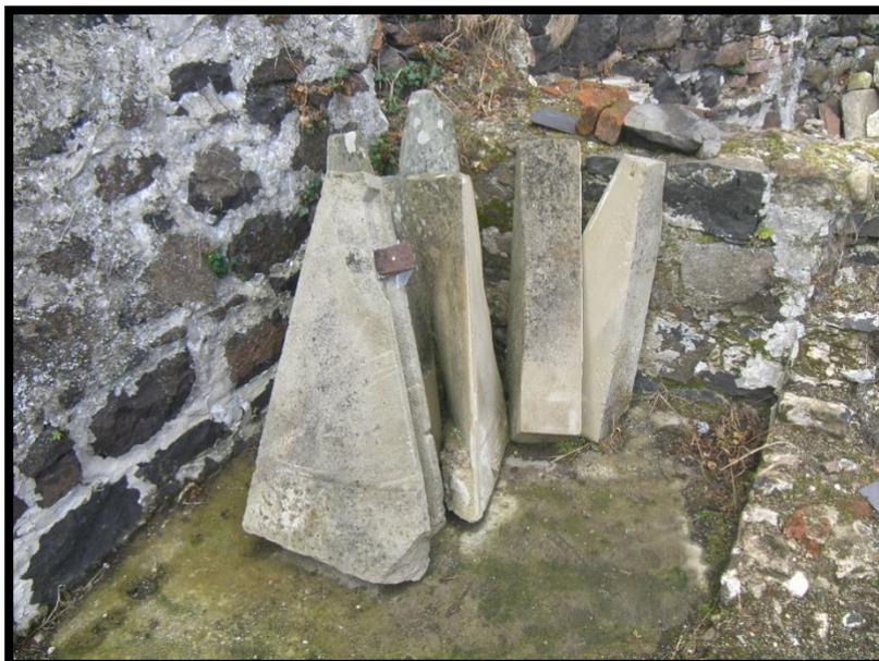
Figure 12: Individual stone steps of a spiral staircase
