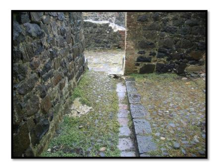
Figure 09: Original cobbled surfaces within buildings in the East Yard
