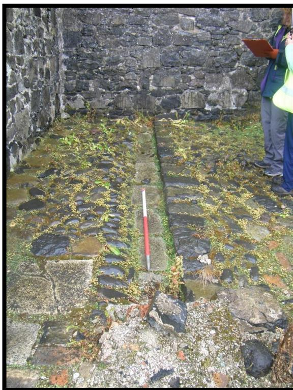
Figure 25: Room 2 from the west, showing drainage channel
